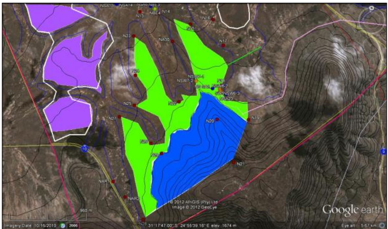
Figure 33. Close-up aerial view of the South Site for the proposed area for the Naauwpoort Solar Energy Facility.
