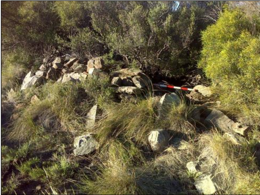
Figure 42. Close-up of the visible dry packed stonewalling foundation.
