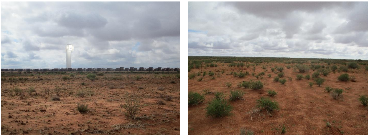
Figure 3 Panoramic view of existing Photovoltaic station towards the south and surrounds.
