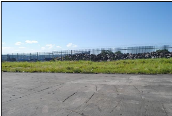
Figure 11: Area 1, facing north (Maitland: 2016)
