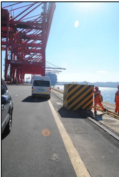
Figure 15: Area 2, facing west (Maitland 2016)
