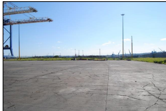
Figure 12: Area 1, facing west (Maitland: 2016)
