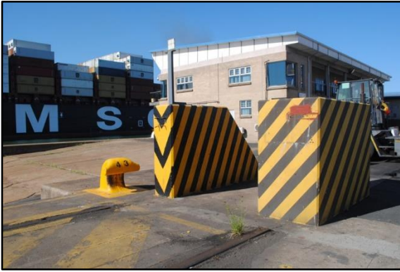
Figure 17: Area 2, facing east (Maitland 2016)
