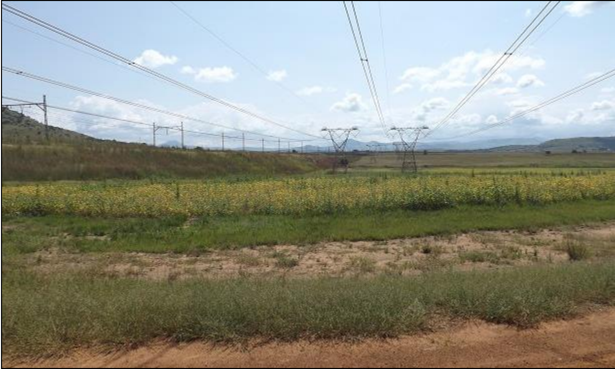
Figure 5: Image showing the railway line embankment, Eskom electricity powerlines and the low-rouned hills to the north.
