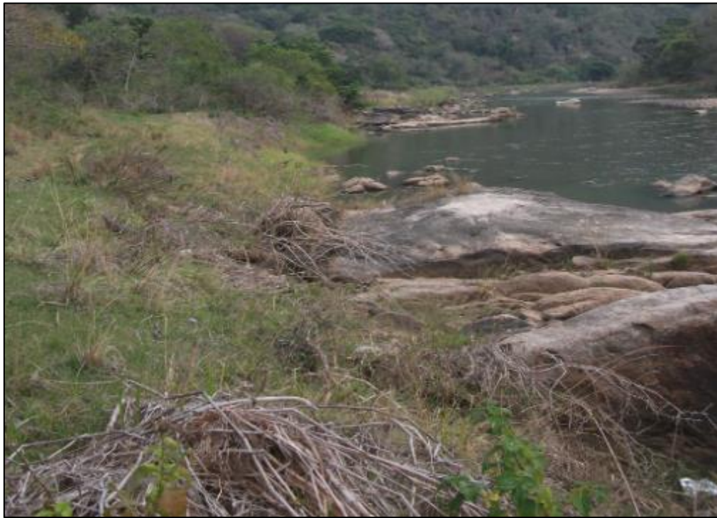
Figure 6: Abstraction works looking up river
