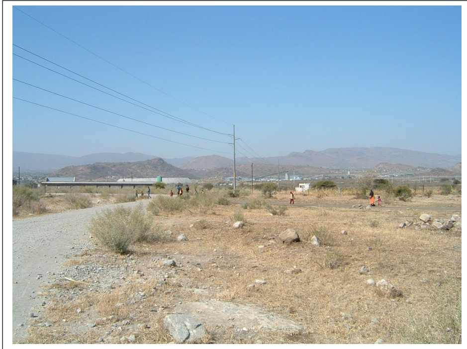
Figure 5- Alternative 01 bends to the west on Clapham 118KT where Marula Platinum Mine is located and then bends through three more consecutive bends in order to run northwards following Eskom's existing 132kV power line (above).
