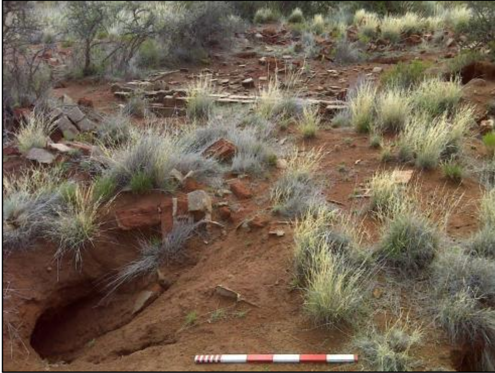
Figure 40. The remains of the foundation of a building.
