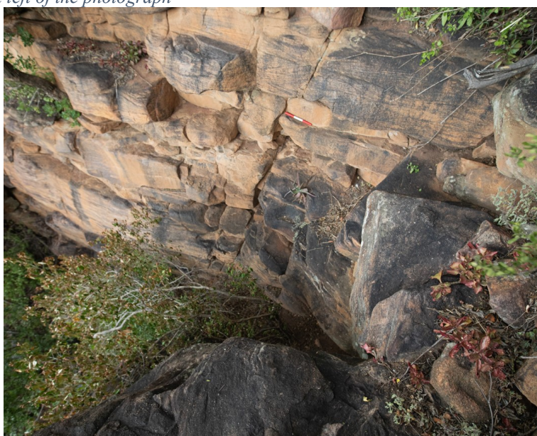
Figure 5. The gulley in which it is suggested that the proposed spiral staircase be placed. The drop down into the gulley from the top of the cliff is about 3 m. The small tree/bush (Croton gratissimus) would need to be removed
