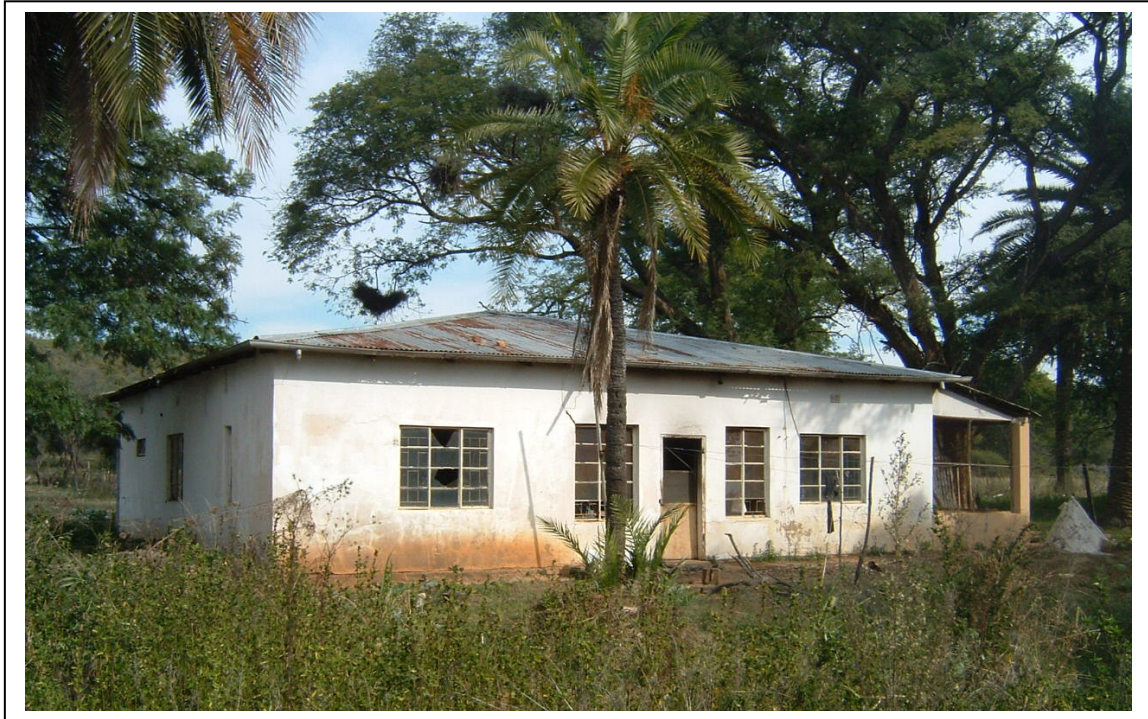
Figure 5- HH01 on Rust De Winter 180JR is a square structure with a pitched corrugated iron roof (above).
