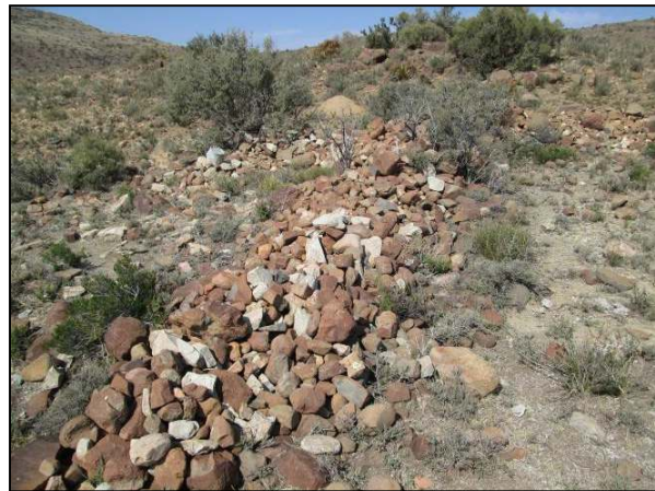
Figure 37: The badly tumbled walls at Site 36. It is likely that the stones forming the outer skins have been removed and reused.
