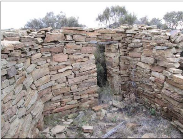
Figure 29: Historical structure at Site 9 showing a doorway with stone lintel.
