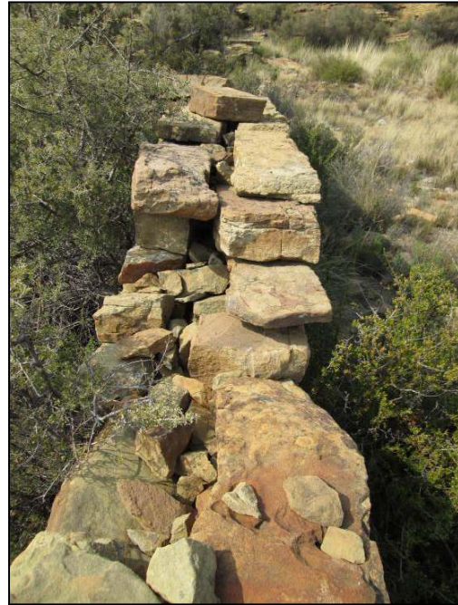
Figure 23: Double skin and rubble fill wall at Site 10 (GPS 069).
