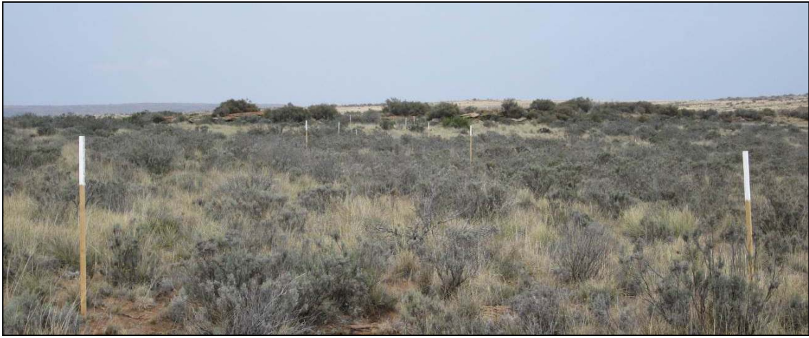
Figure 9: The survey pegs indicating the road layout.
