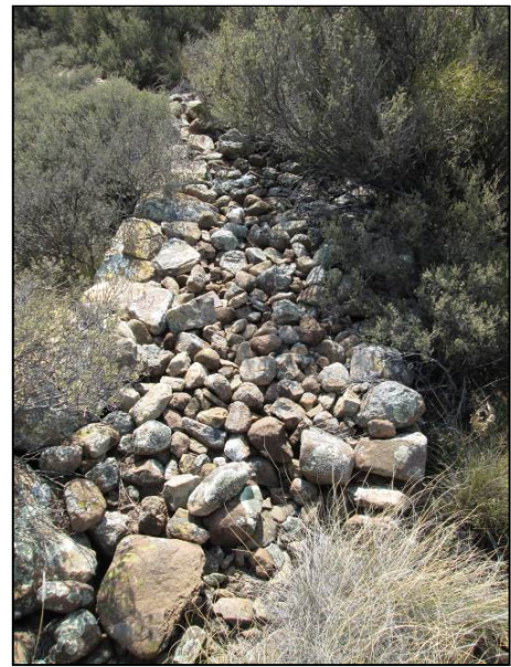
Figure 33: The extra thick wall (c. 1.2m) at Site 6. This wall is also made of two skins with a rubble fill.
