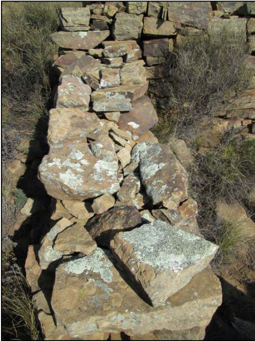
Figure 22: Double skin and rubble fill wall at Site 6 (GPS 017).
