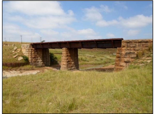
Figure 22: Sandstone bridge at Feature 10.
