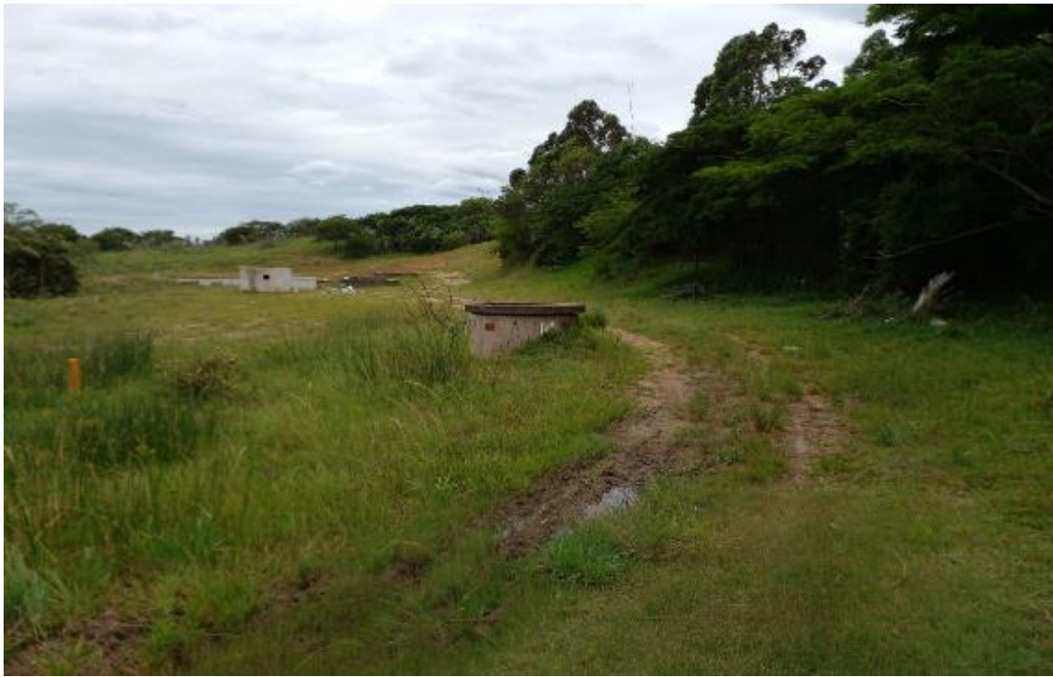
Figure 18: Existing infrastructure and access road
