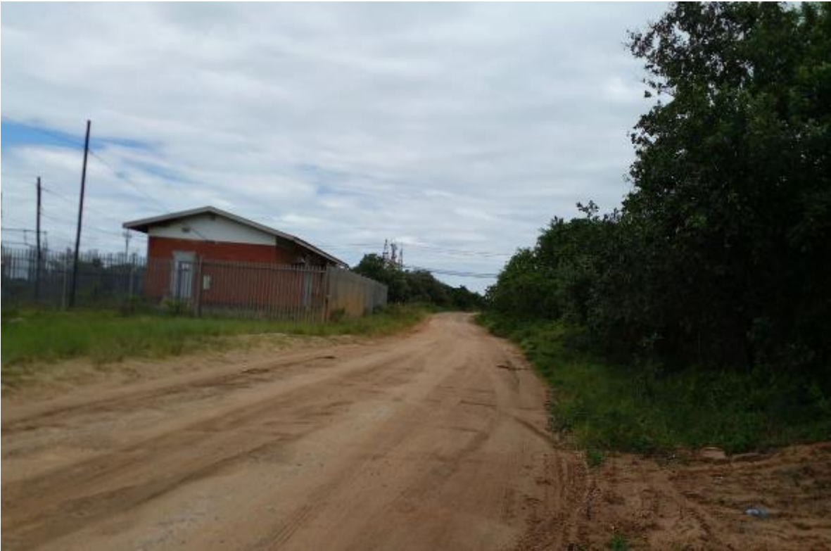
Figure 15: Mini-substation between road and railway line
