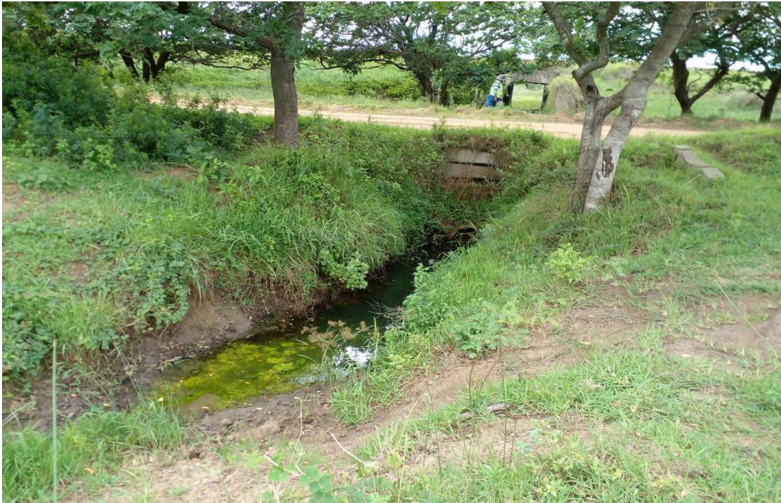
Figure 9: Stormwater outlet
