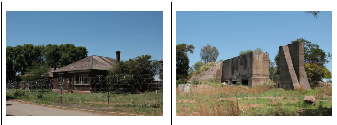
Fig. 4. Remains of mining related structures in the region.
