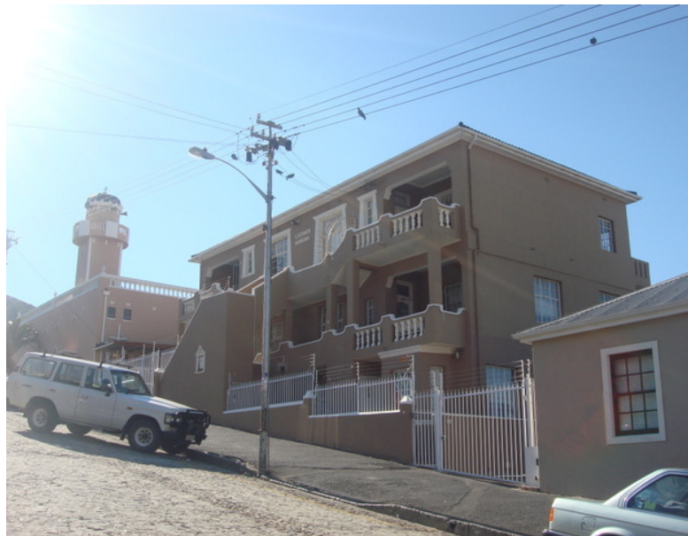
Figure 7: View in a northerly direction with Leeuwen Mansions in the foreground and Nur-el-Huda in the background
