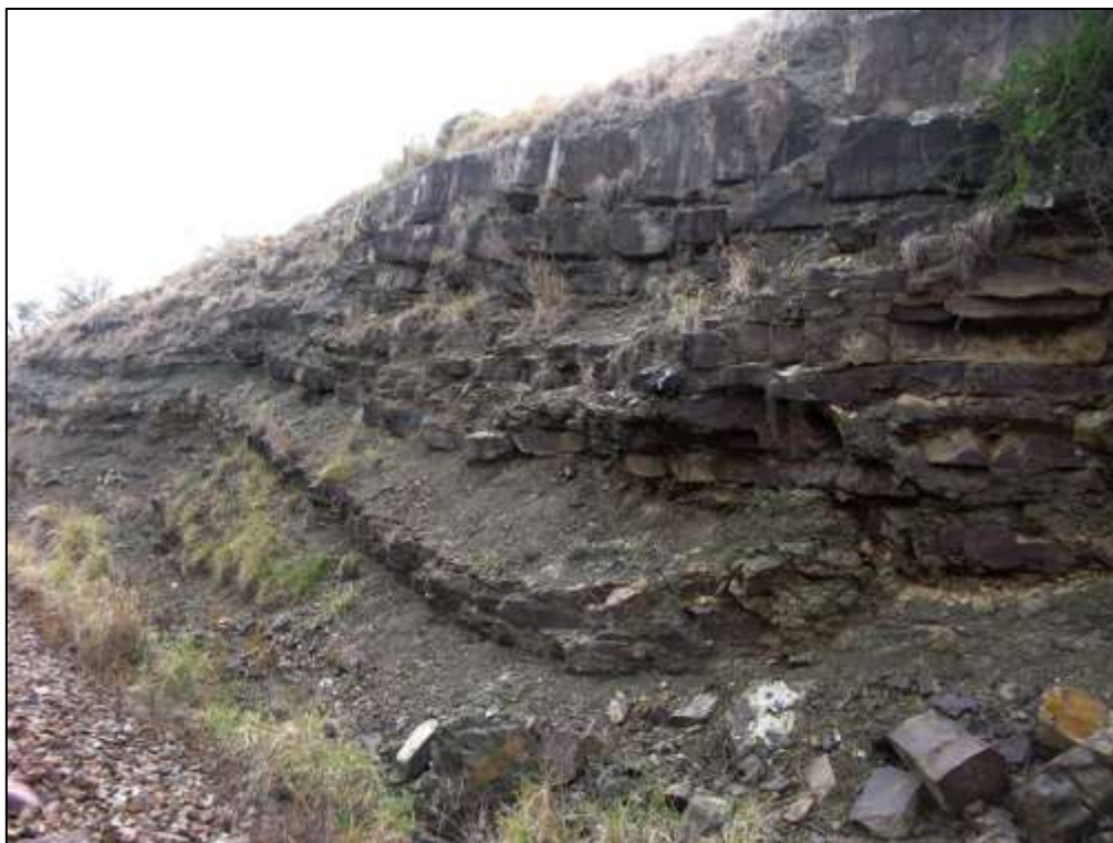
Figure 28. Thin- to medium-bedded channel sandstones with intercalated mudrock horizons overlying the main mudrock package seen in Figures 25 & 26 above, northern end of railway cutting on Request 71 (Loc. 386).
