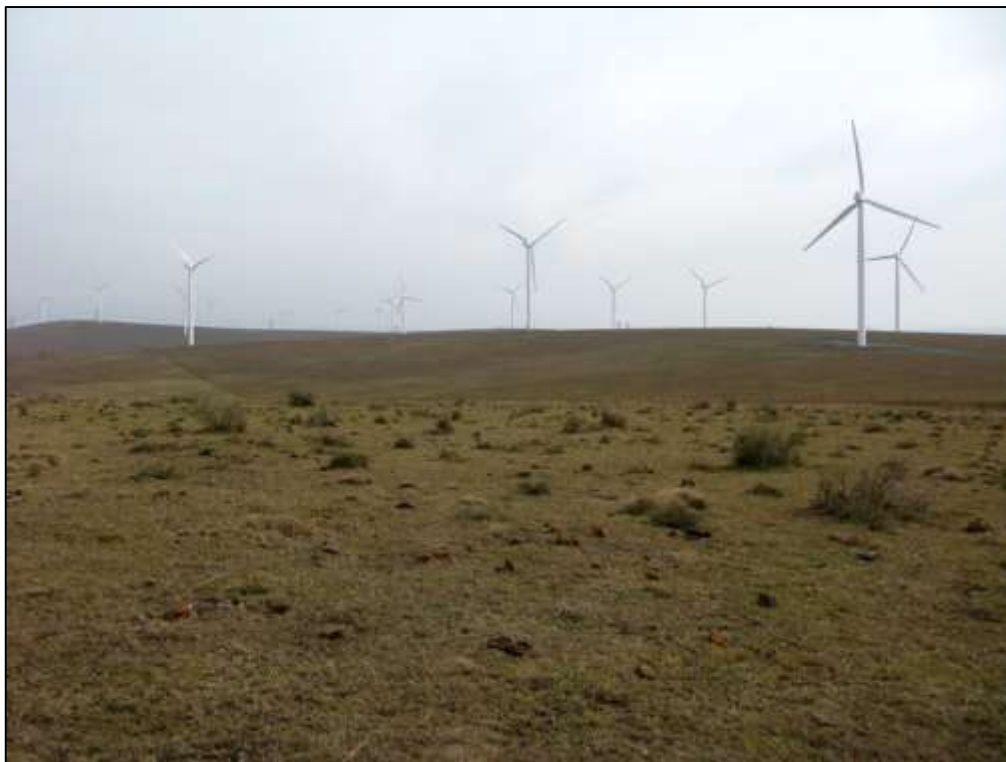
Figure 5. Typical upland ridge terrain in the north-western sector of the Nxuba Wind Farm project area showing gentle, grassy slopes and lack of bedrock exposure (Request 71, close to Loc. 389).
