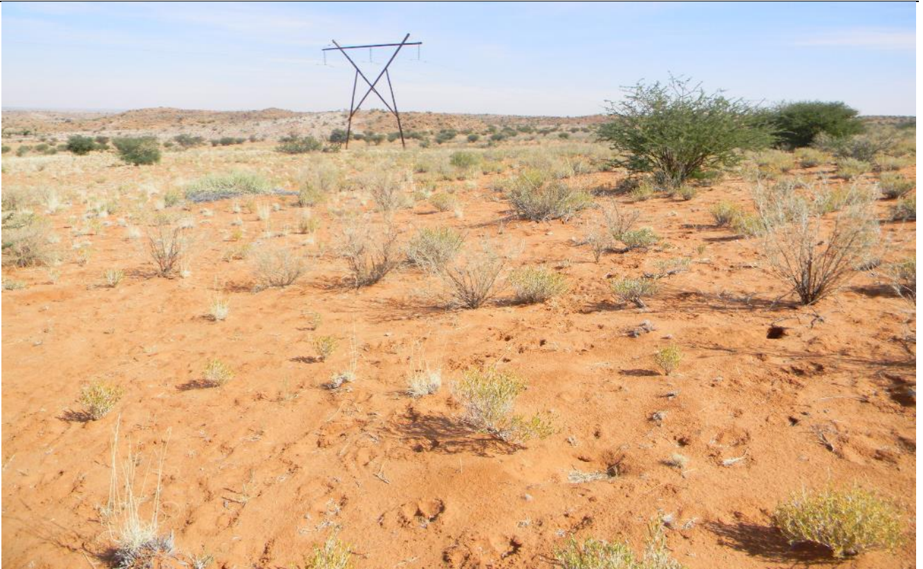
Plate 15: Photo 15: View of existing infrastructure near terminal position for Alternative 2 powerline deviation route (Photograph © by Author 2017)
