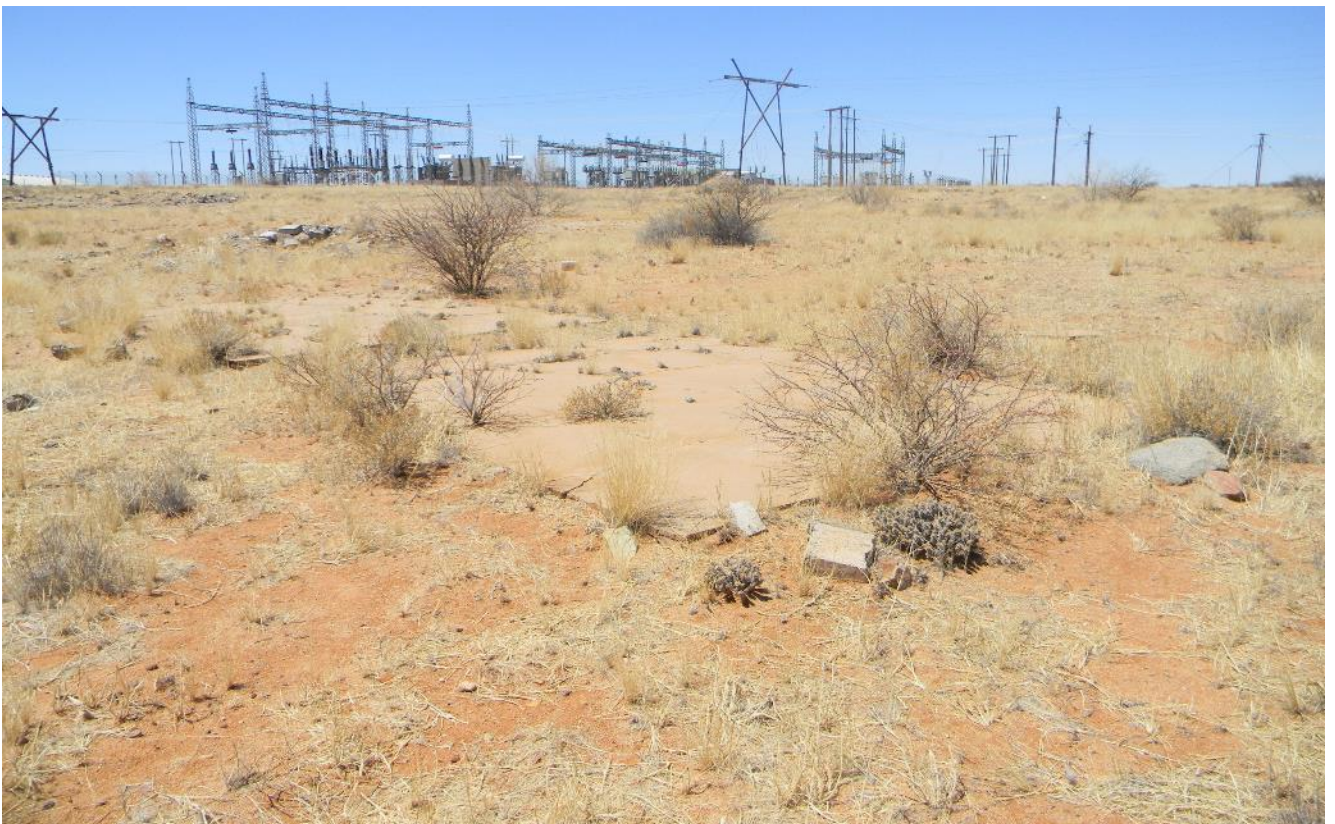
Plate 22: Photo 22: View of Taaipit Substation where the proposed powerline development will terminate (Photograph © by Author 2017). Note remains of campsite dwellings near substation.
