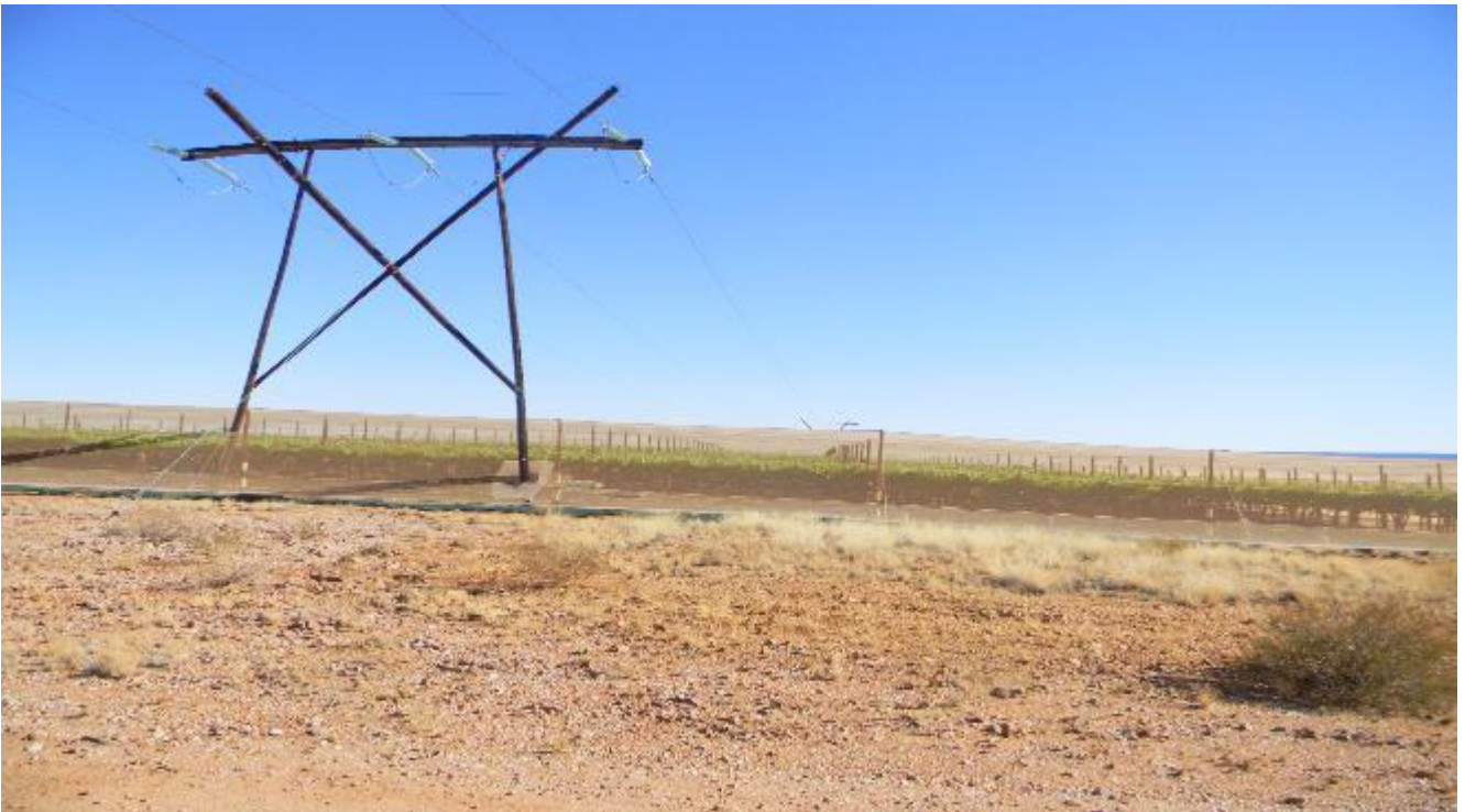
Plate 2: Photo 2: View of wooden structures to be replaced by steel monopole structures (Photograph © by Author 2017). Note that the powerline cuts through vine yards.
