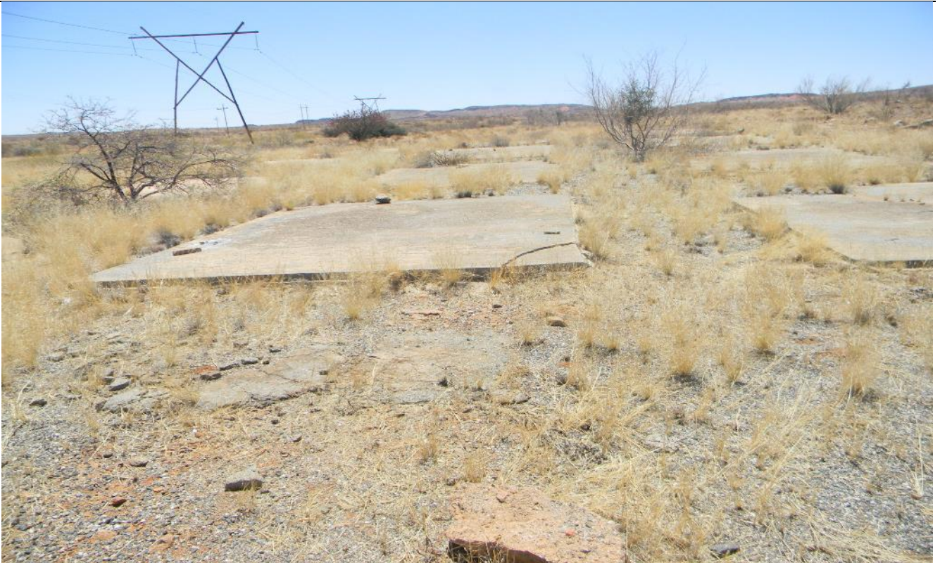
Plate 21: Photo 21: View of tower position where the proposed deviation will be connected (Photograph © by Author 2017).
