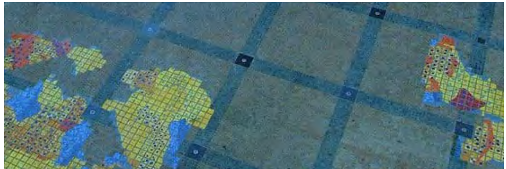
Insertion of coloured paving in designated areas
