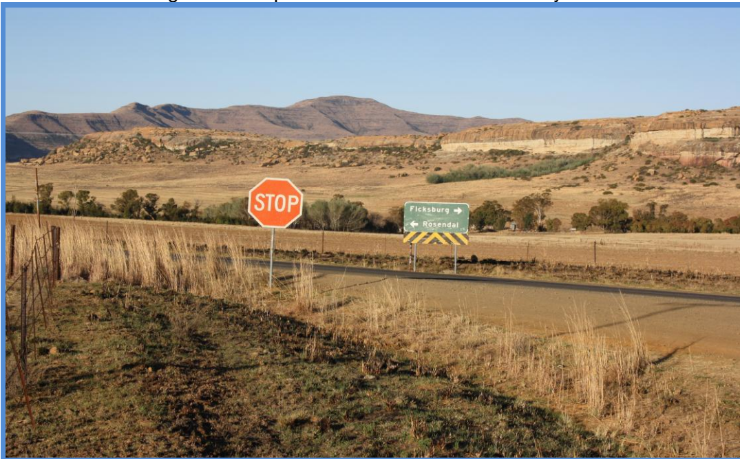
Figure 4: View of the main tarred road and gravel intersection at a distance R70 from Rosendal to Ficksburg, the proposed pipeline have been earmarked parallel the tarred road still on the inside of the farm boundary fence.
