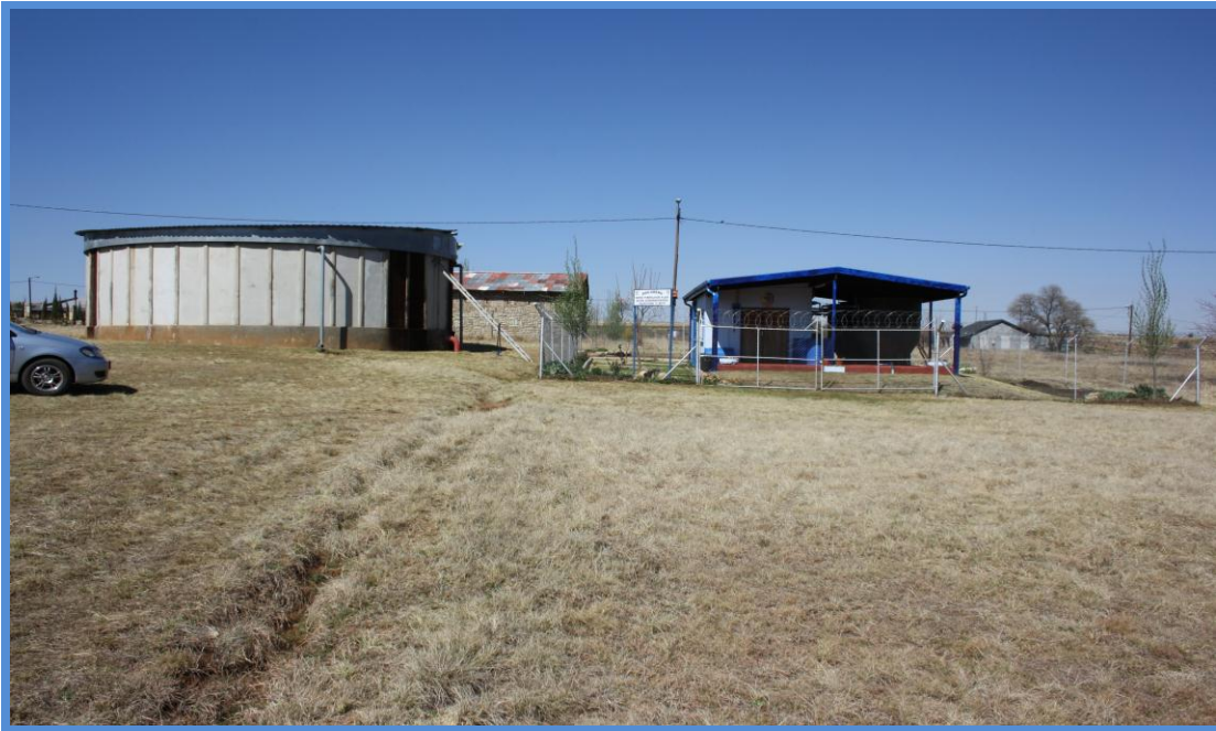
Figure 6: View of Rosendal water purification plant characterized by concrete reservoirs and water treatment house.
