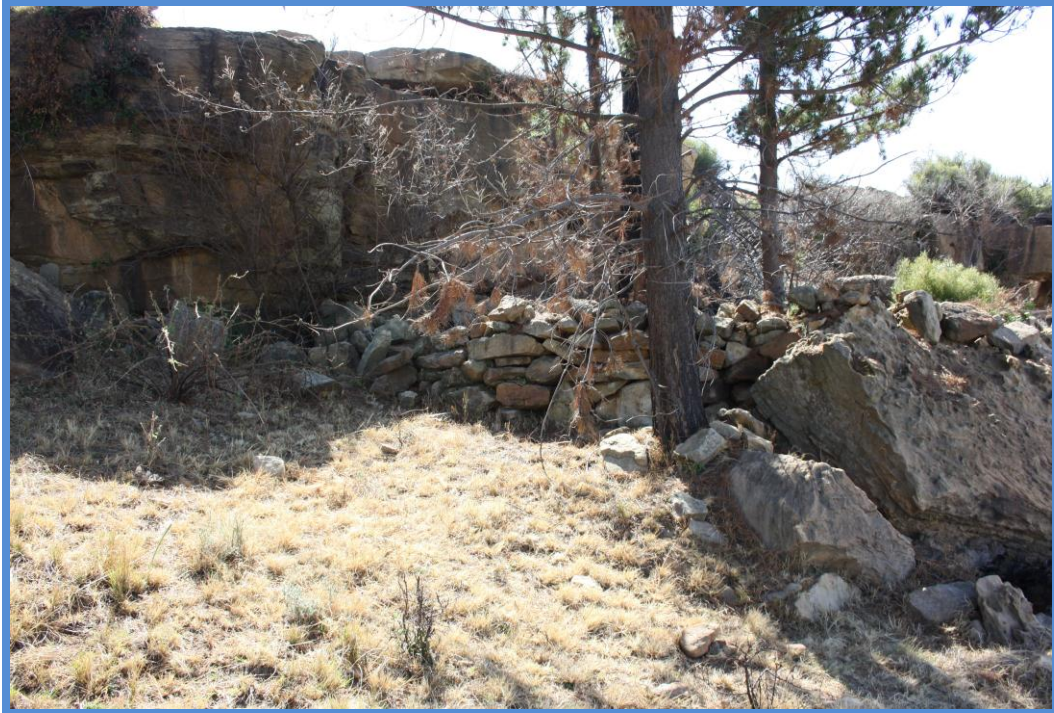
Plate 16: Section of the stone wall enclosure constructed against the boulders and Cliff overlooking the Meulspruit.
