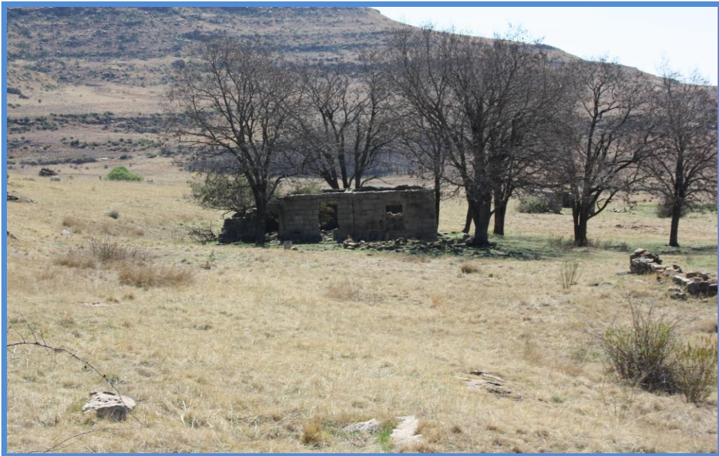
Plate 08: View of the homesteads indicated by a house and associated out buildings Constructed out of sandstone blocks without and cements mixture.
