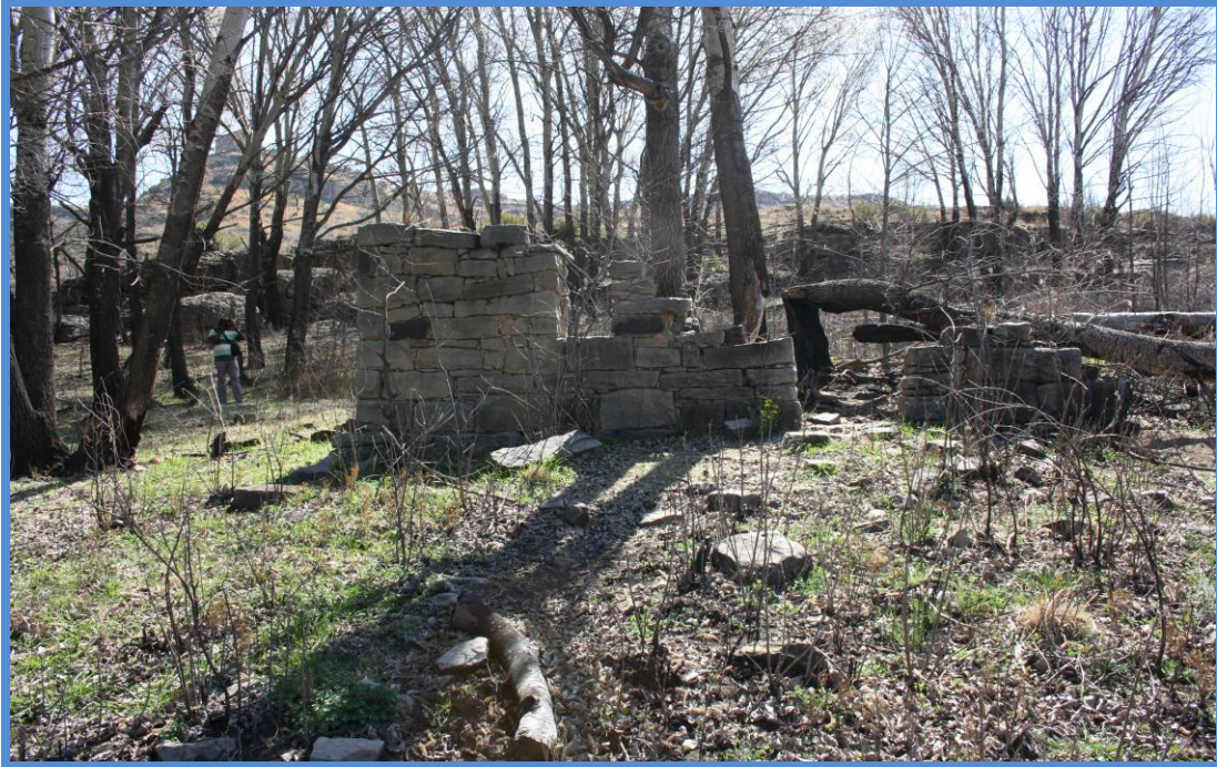
Plate 14: View of the homestead represented by dilapidated house
