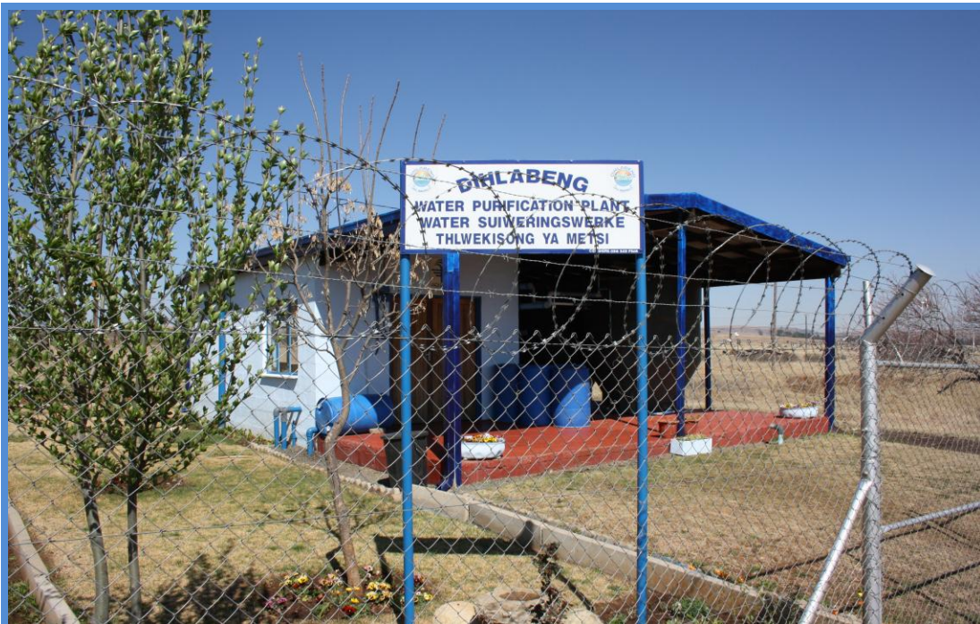
Figure 7: View of the existing water treatment plant
