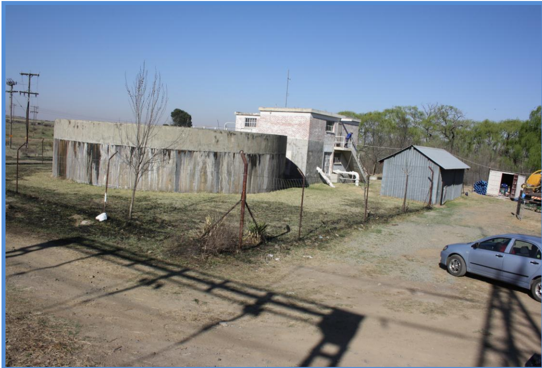
Figure 8: View of the Senekal water treatment plant, the area is located at Senekal industrial site.
