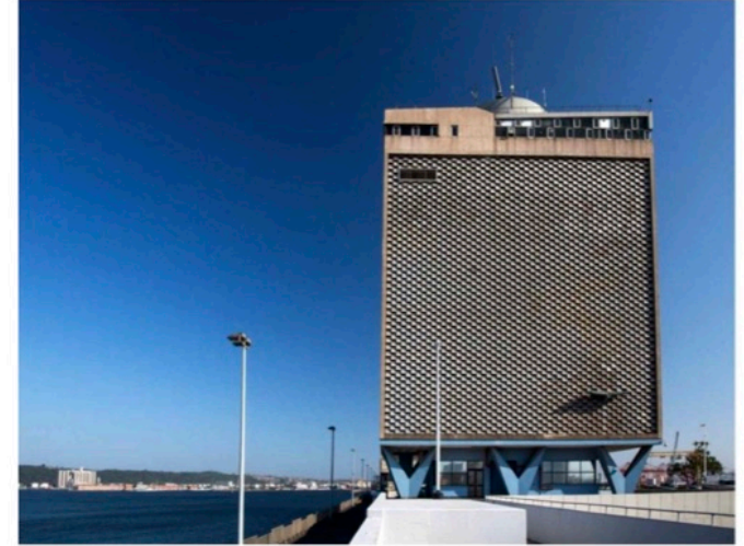
Durmarine, The Galleon sculpture missing
