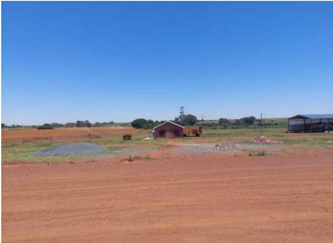
Figure 12: Another general view of the area and some of the modern structures located here (courtesy AB Enviro).
