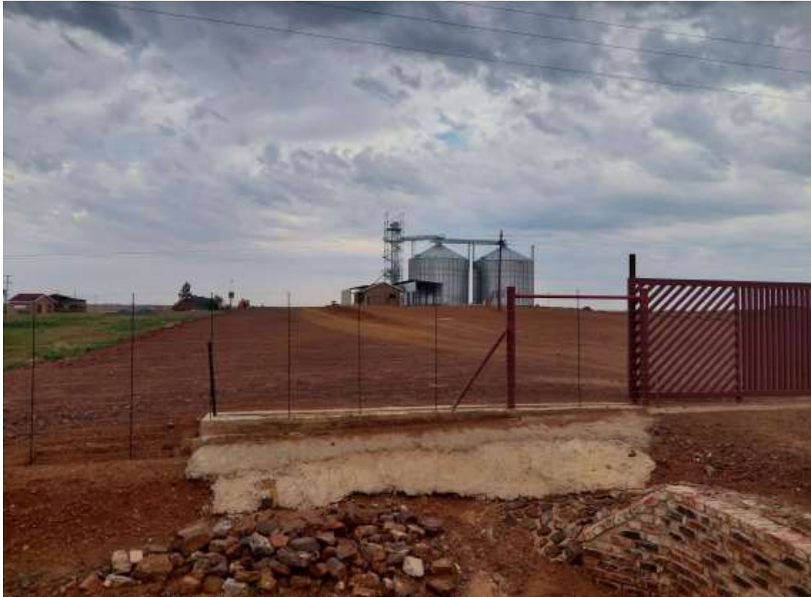
Figure 10: A view of the existing Silos and structures at the NWK Waagkraal site (courtesy AB Enviro).
