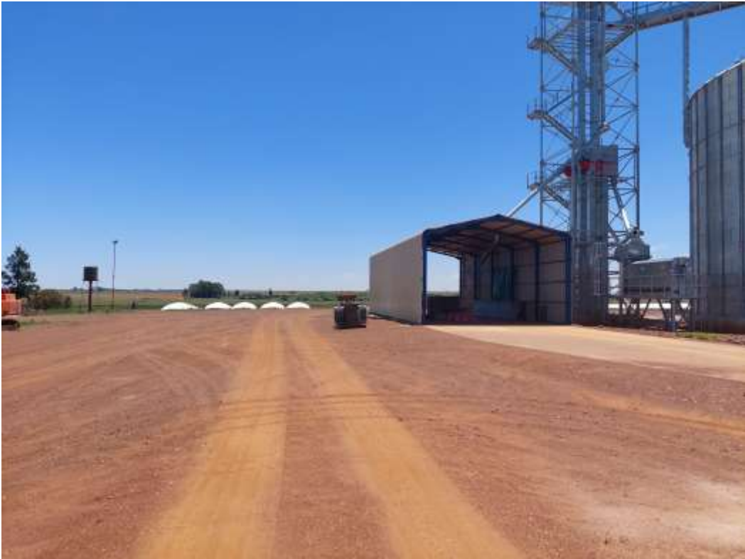
Figure 13: View of some structures associated with the existing Silos (courtesy AB Enviro).
