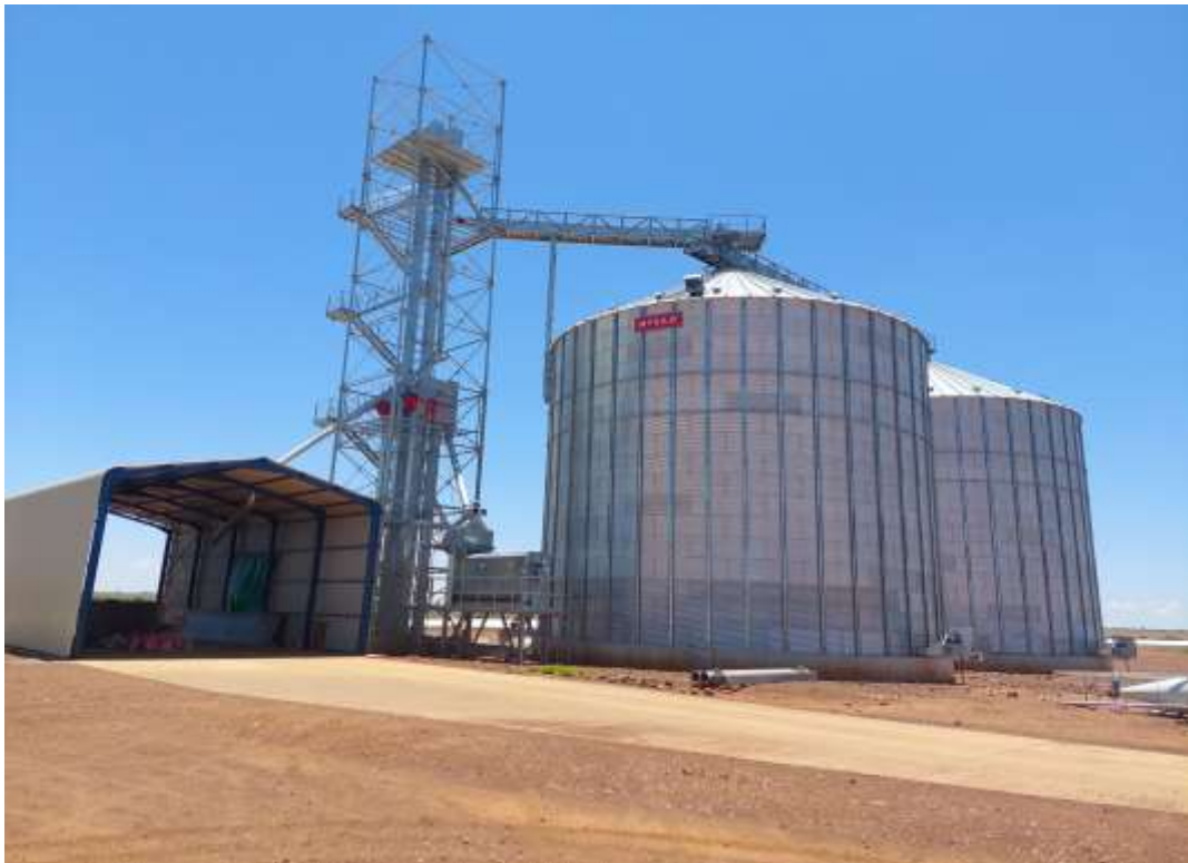
Figure 14: Closer view of the Silos (courtesy AB Enviro).
