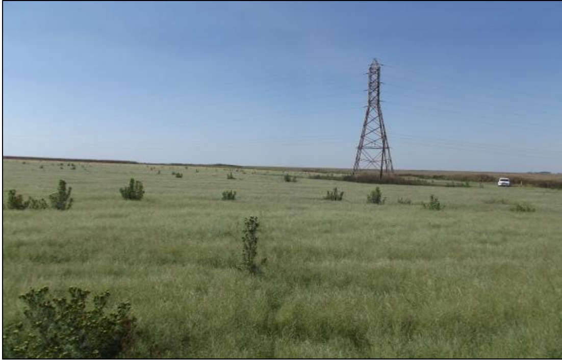
Fig. 27. Site SO 4. Looking towards the South-east from where the planned powerline will start.
