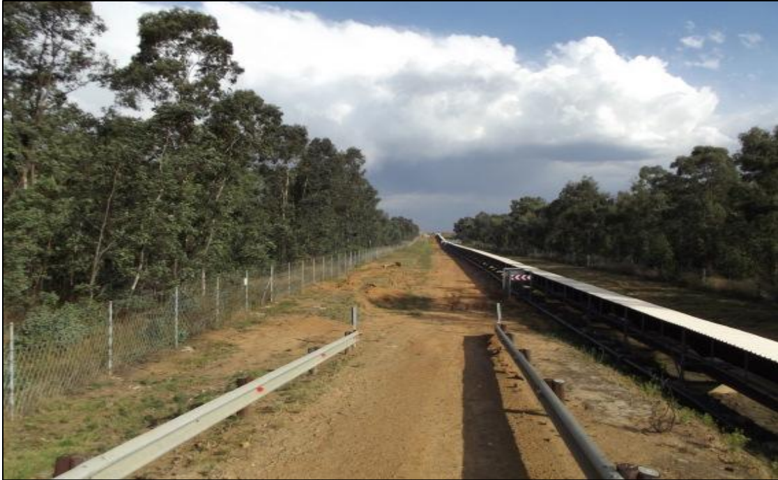
Fig. 47. Site SO 15. Looking in a Southern direction along the proposed route of the new powerline (alternative 1&2).
