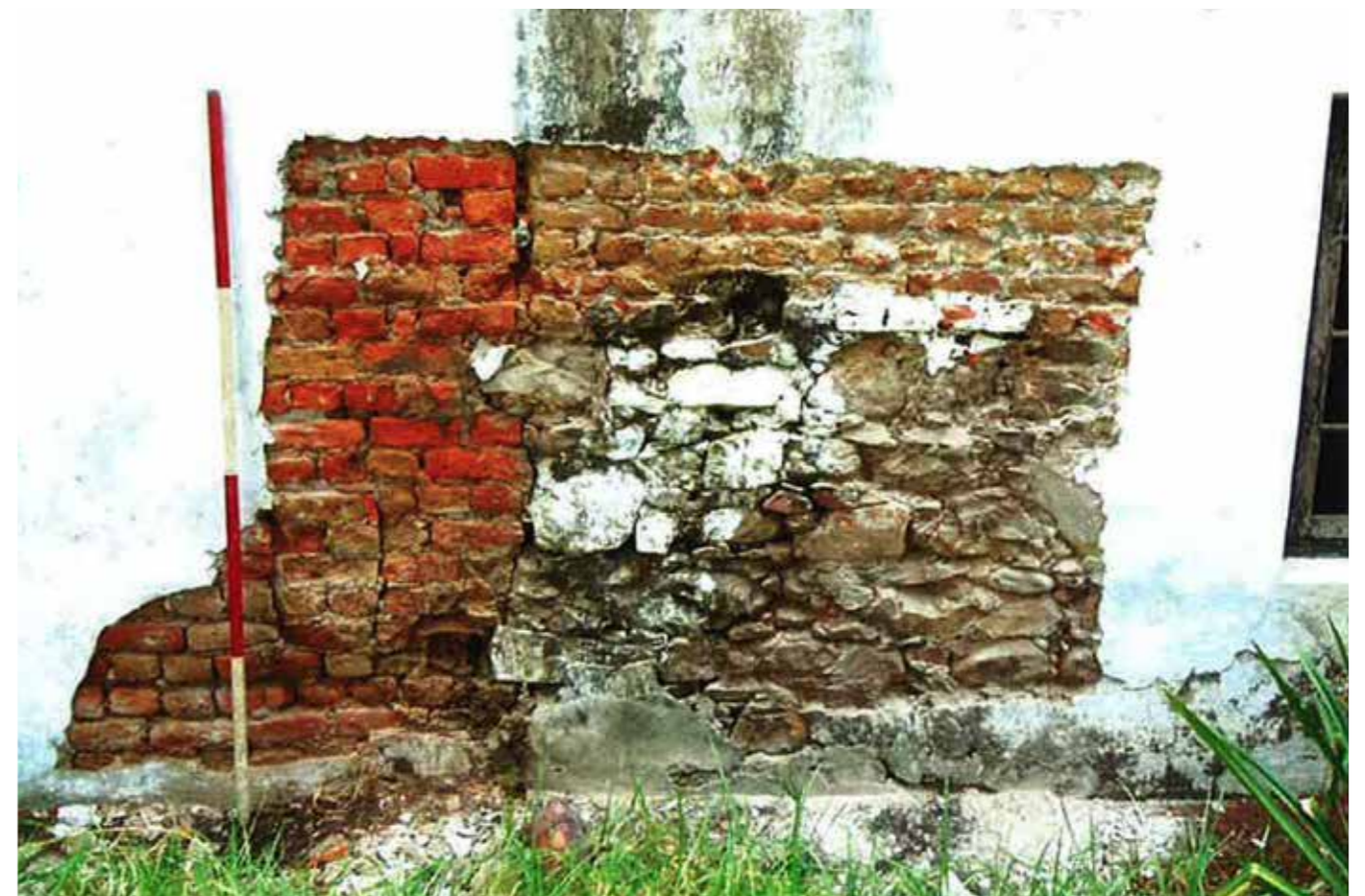
Figure 19. Building morphology: stone walling of phase 1 meets brick walling of phase 2 c1780+. (Image: Vos 2011)
