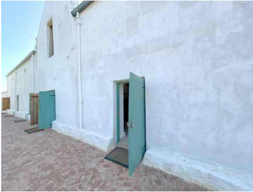
Careful intervention with stone plinth and thresholds on front/north elevation
