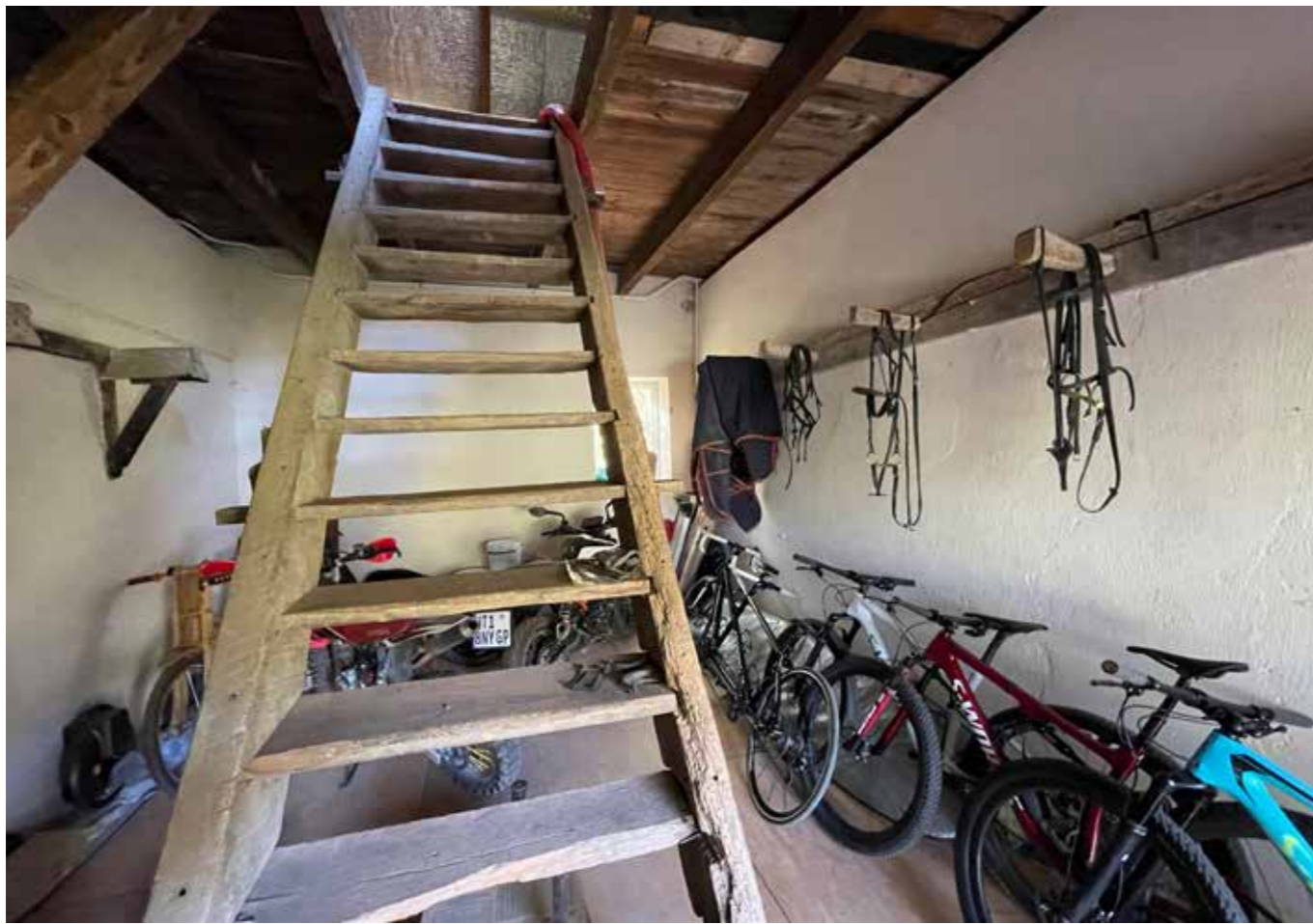
Figure 13. Central entrance space with access to attic and intact artefacts c1900 (Image: RSA 2023)
