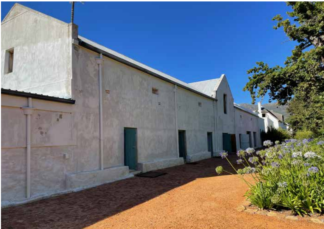
Figure 5. East end gable and front facade 2018 (Image: RSA)
