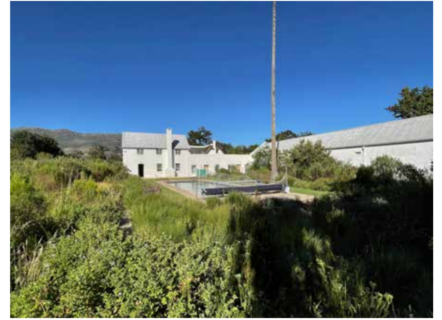
Rear/south werf garden area: has the capacity to comfortably absorb a new intervention
