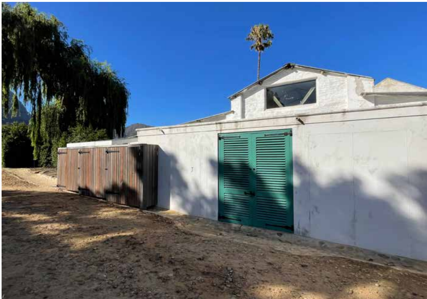
Figure 14. North east end wall of barn (Image: RSA 2023)
