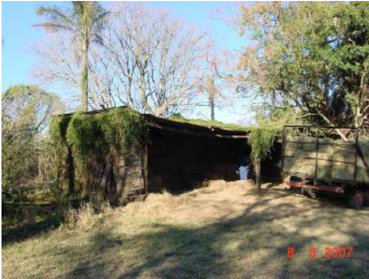
Fig 19: Showing shale barn from the north
