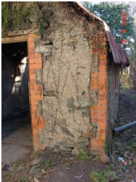
Fig 26: showing construction of cool-room
