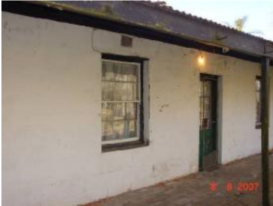
Fig 4: view of main veranda to the south
