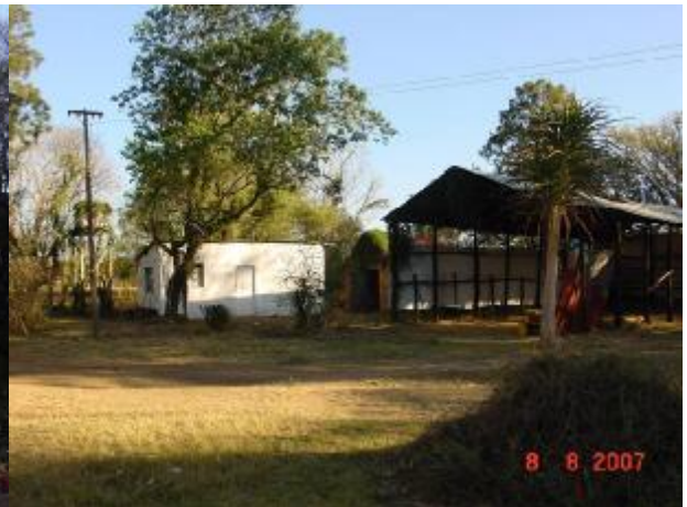
Fig 25: group showing fly-ash rammed building on left and cool room behind shed structure.
