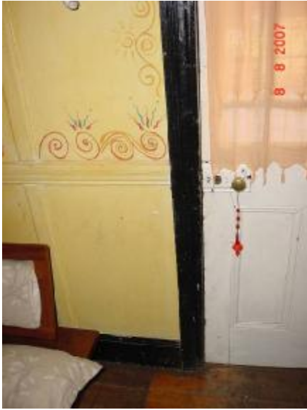
Fig 10: door from main room to east veranda- note the chair rails in the paneling
