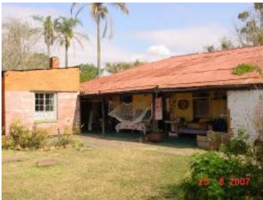
Fig 17: showing house from east
