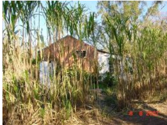
Fig 21: Barn from the north
