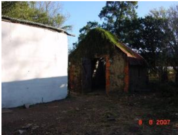
Fig 24: entrance to cool-room building
