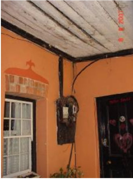
Fig 15: back veranda-entrance to bathroom
