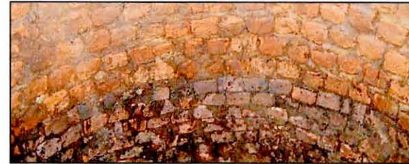
Plate 9: Close-up photograph showing the transition between the orange and the pink/brown bricks used in the walls of the well.
