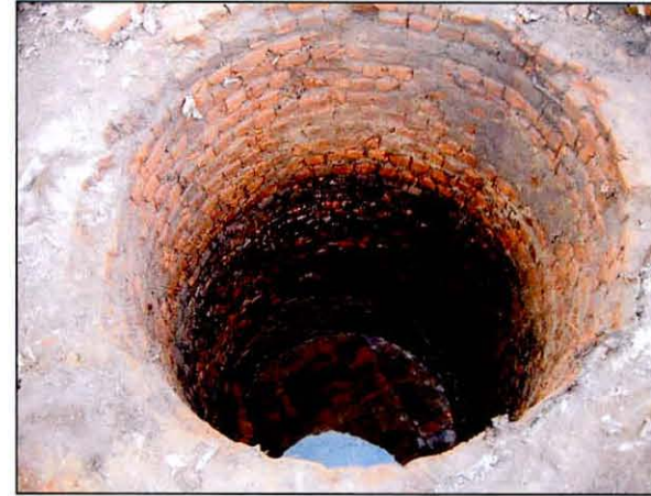
Plate 8: The interior of the well after completion of the excavation.
