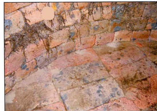
Plate 11: The base of the well showing the tightly packed brick paving extending beneath the side walls.
