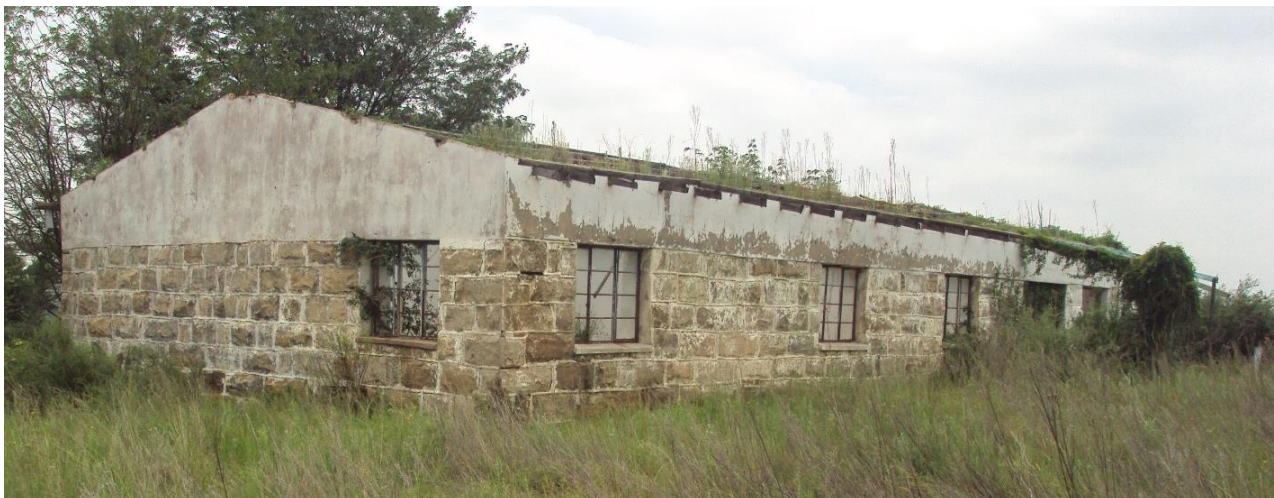
Figure 25: View of the rear elevation of the main farmhouse, showing the sandstone construction material
