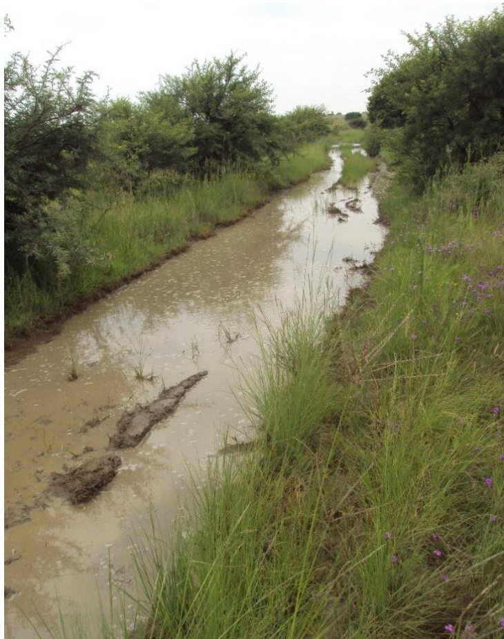
Figure 11: View of a section of flooded road in the southern section of the project footprint
