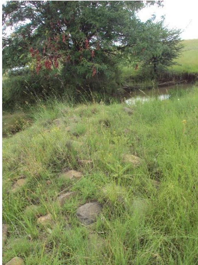
Figure 48:: View of southern end of the stone wall remains, LILO-04
