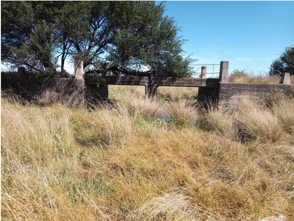
Figure 39: View of concrete road bridge/ culvert at Os3-05
