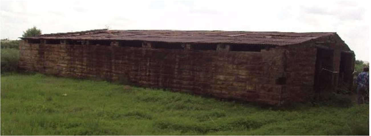
Figure 52: View of historical barn/shed building (LILO-05B)
