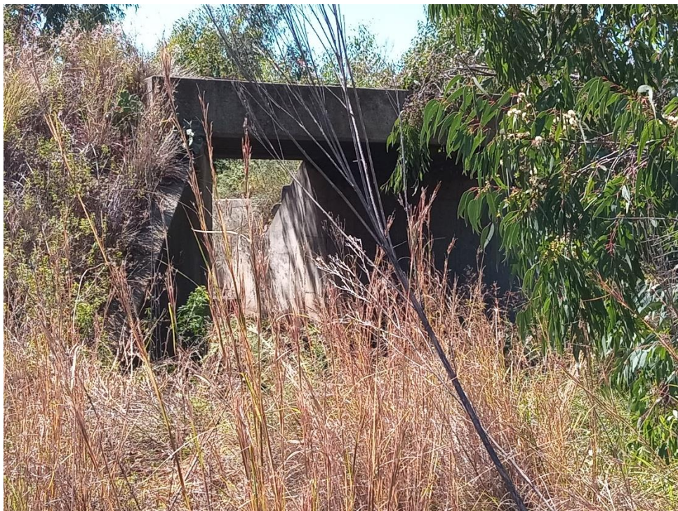
Figure 38: View of the concrete railway culvert at Os3-04
