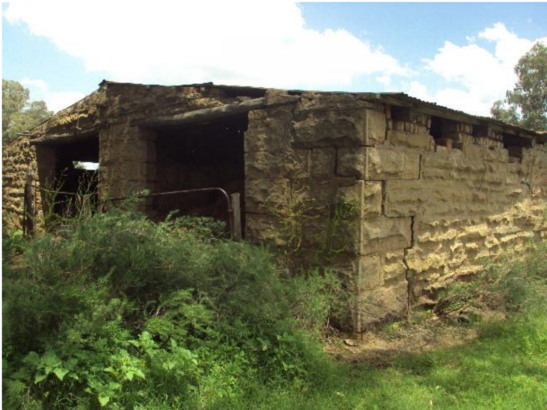
Figure 53: View of entrance to historical barn/shed, showing sandstone construction material
