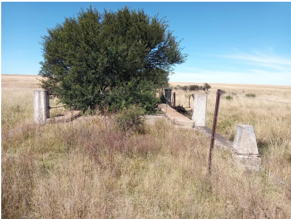
Figure 40: View of the top of the disused road bridge/culvert
