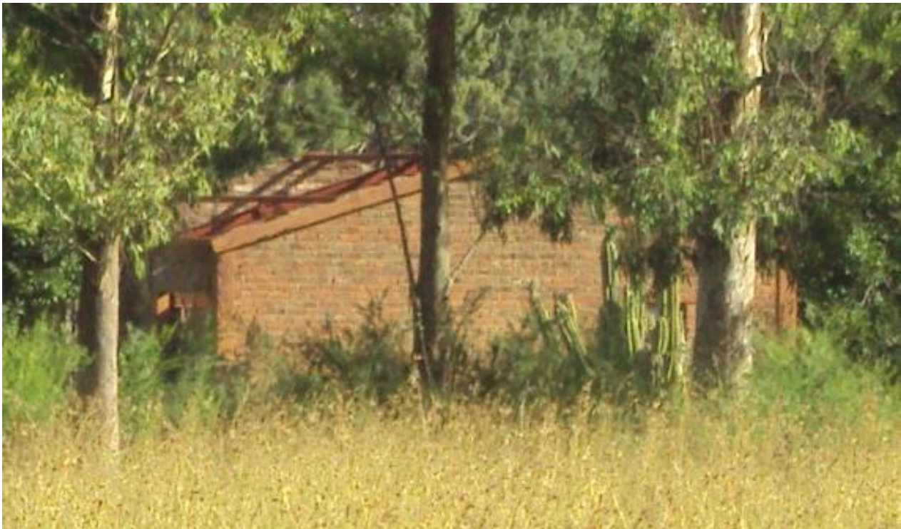
Figure 30: View of associated brick outbuilding, with the roof missing
