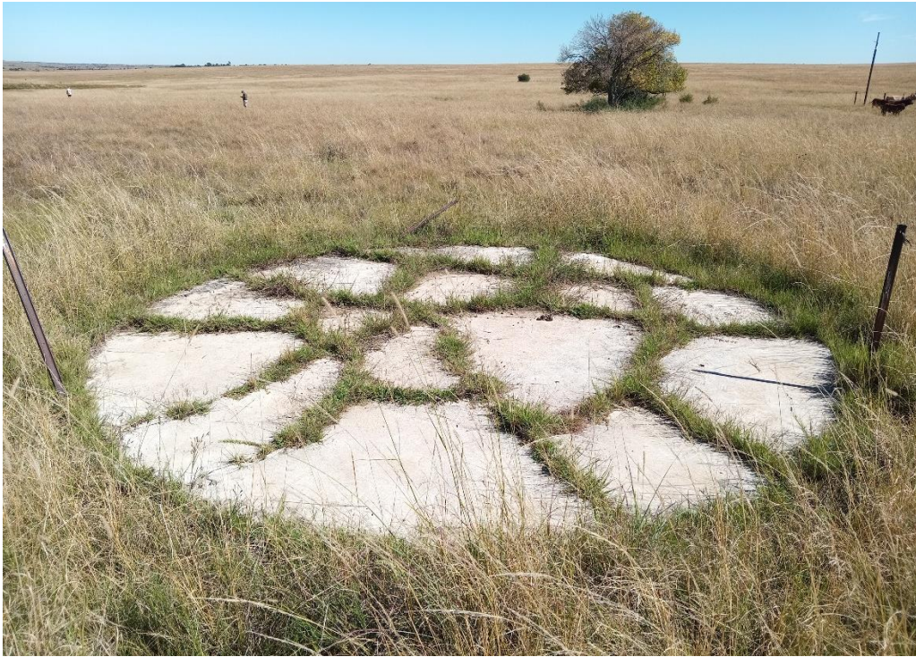
Figure 34: View of circular cement foundation at Os3-02
