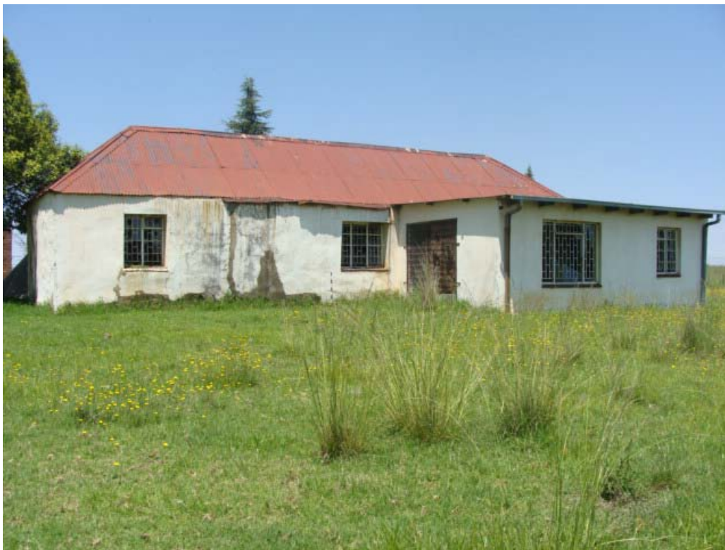
Figure 8 Northern façade of the farmstead.
