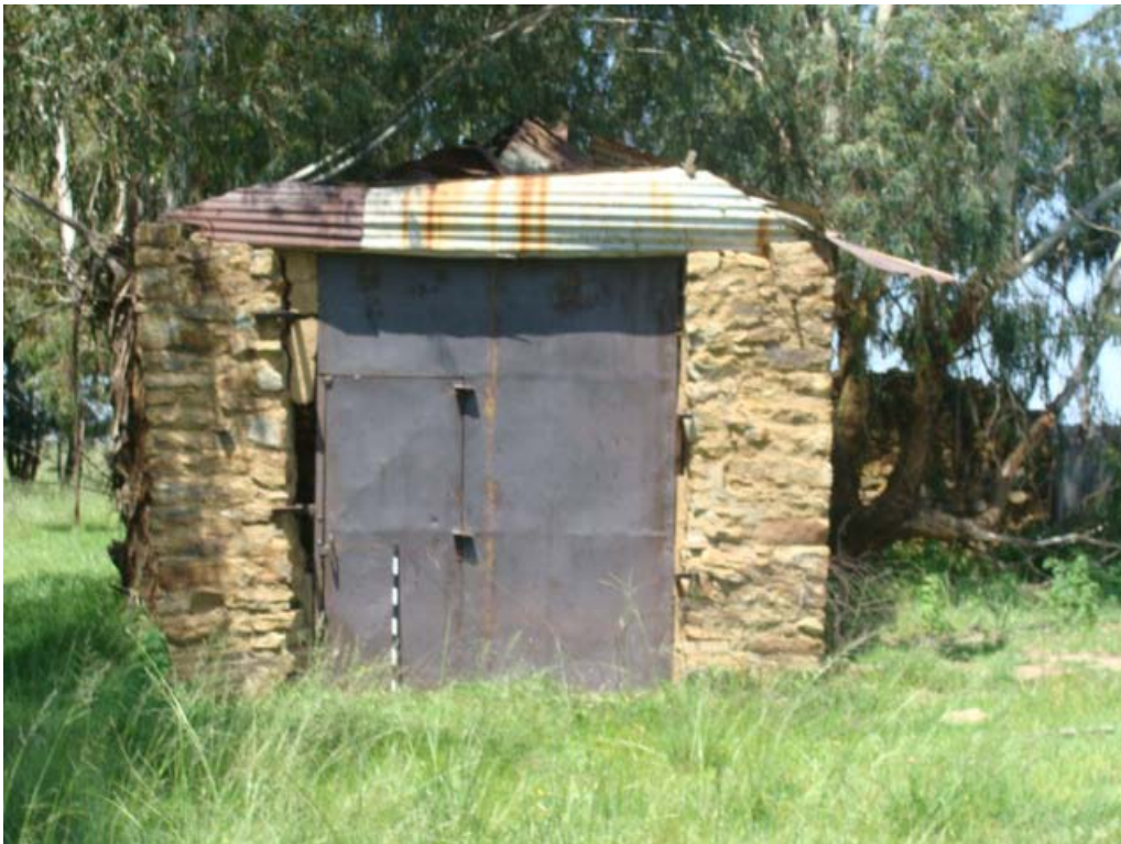
Figure 7 Western façade of the wagon house.
