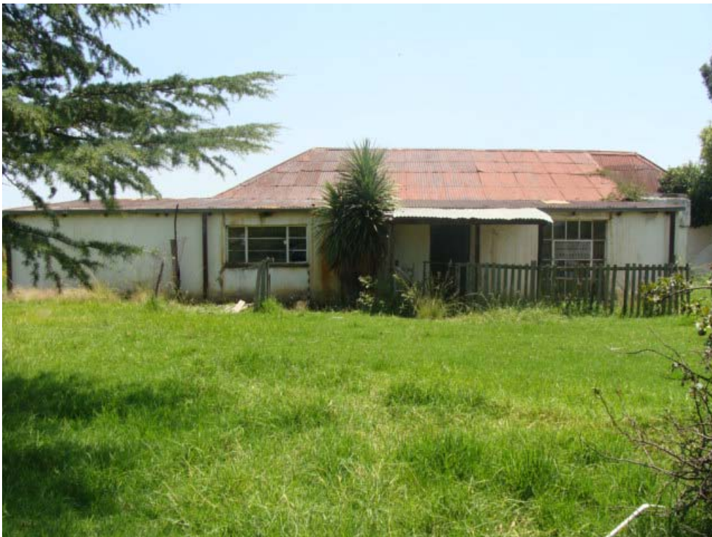
Figure 10 Southern façade of the farmstead.
