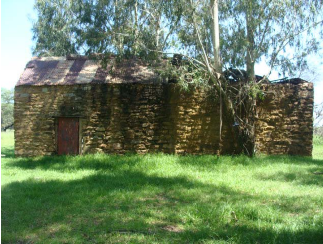
Figure 4 Northern façade of the wagon house.
