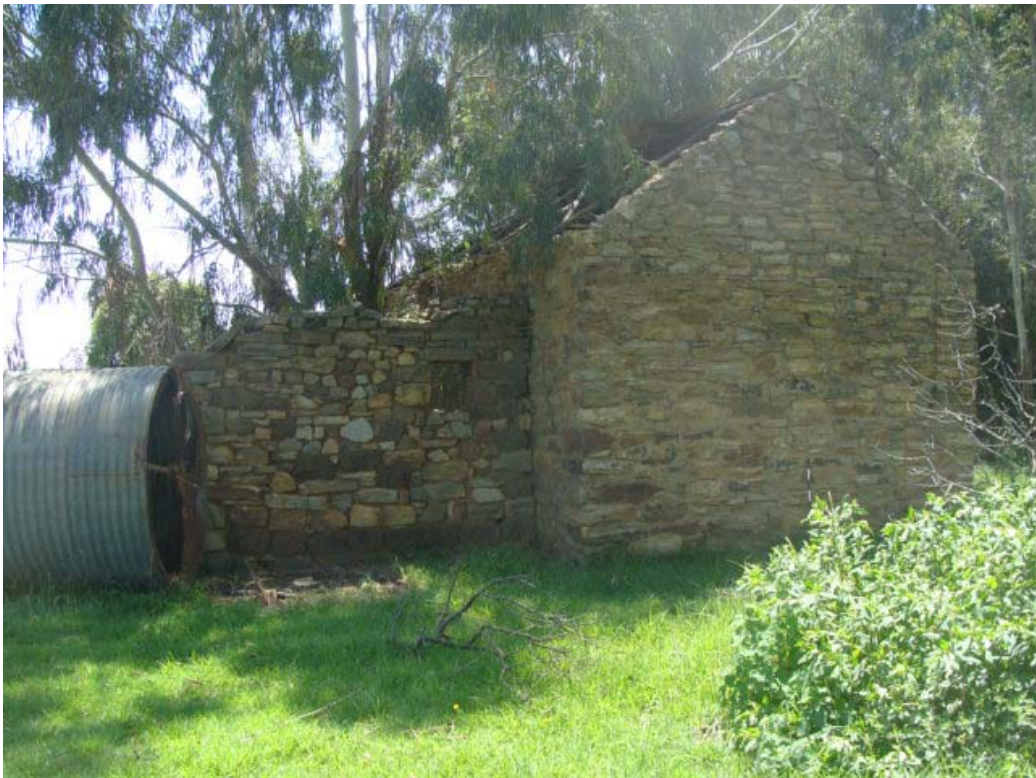
Figure 5 Eastern façade of the wagon house.
