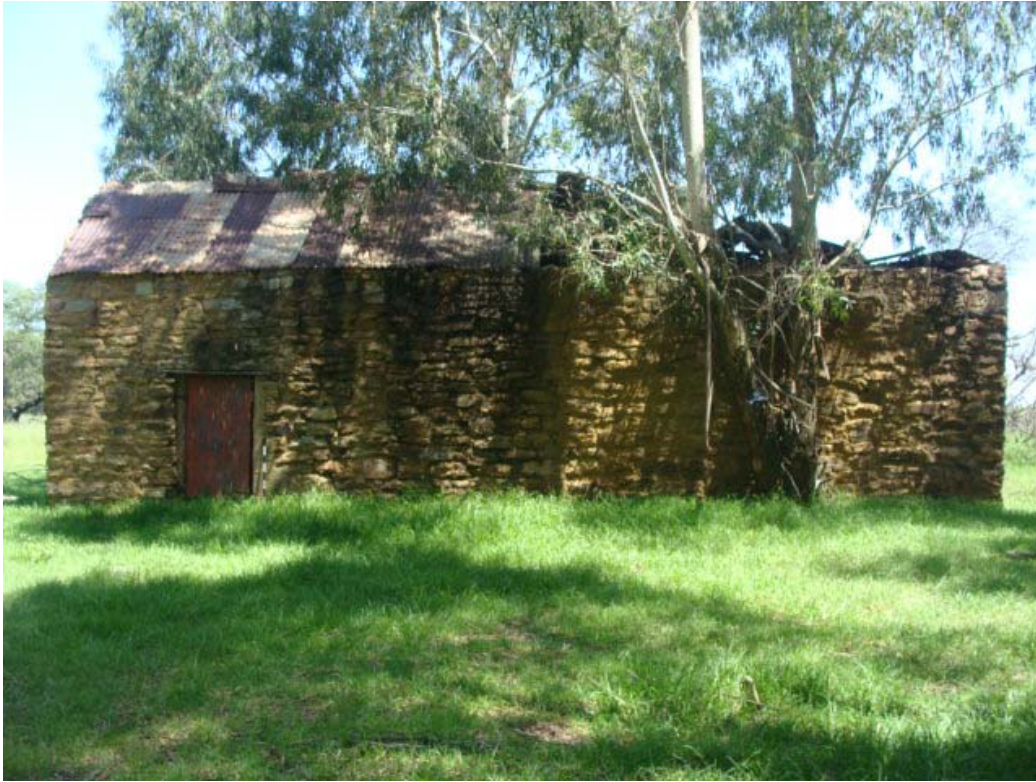
Figure 4 Northern façade of the wagon house.
