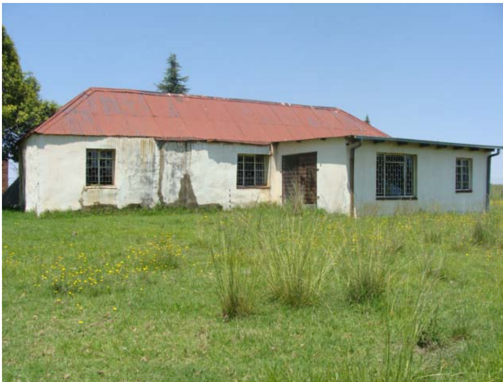
Figure 8 Northern façade of the farmstead.
