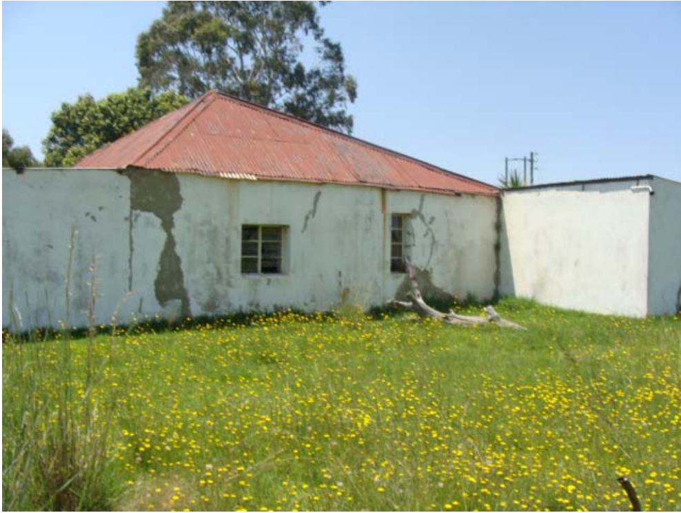
Figure 11 Western façade of the farmstead.
