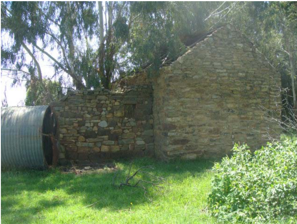
Figure 5 Eastern façade of the wagon house.
