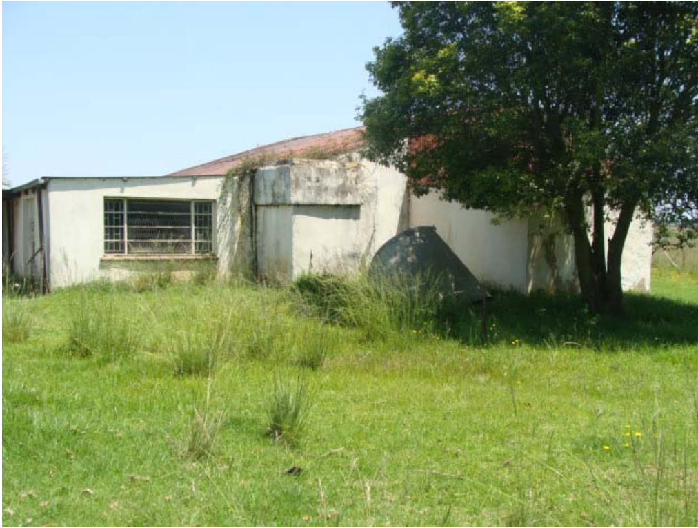
Figure 9 Eastern façade of the farmstead.
