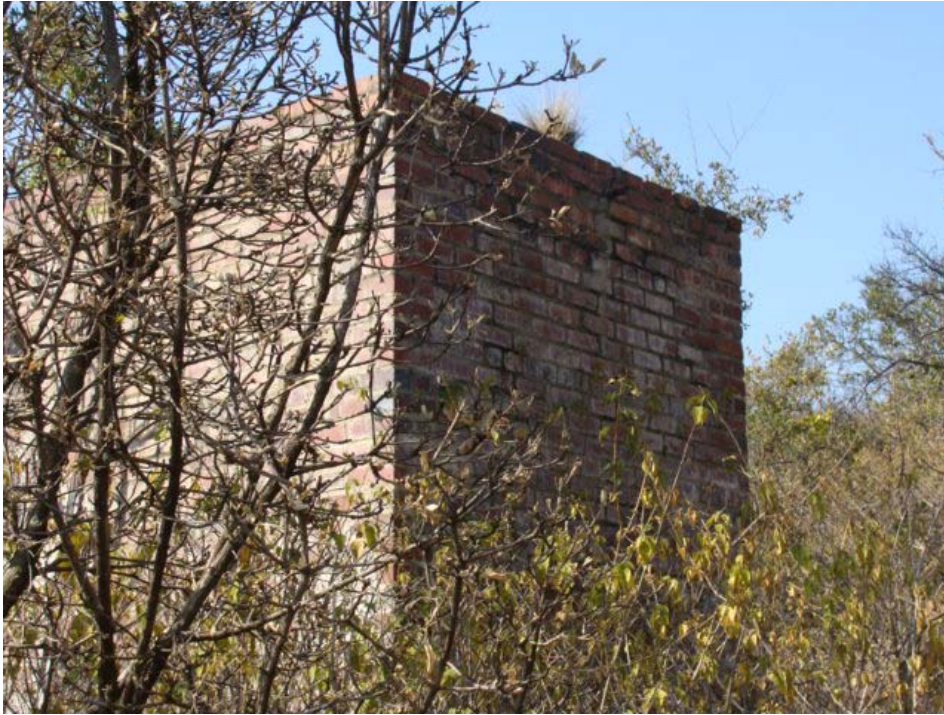
Figure 12 Brick building which served as base for a water tank.
