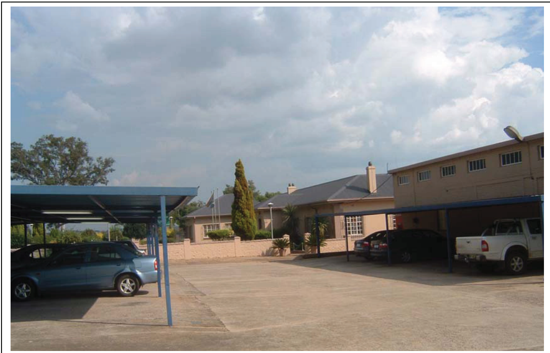
Figure 3- The administrative offices of X Strata Coal Tweefontein Division include several structures which qualify as historical buildings as they approach an age of sixty years (above).
