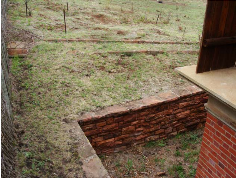
Figure 24 Another view of site no 7.
