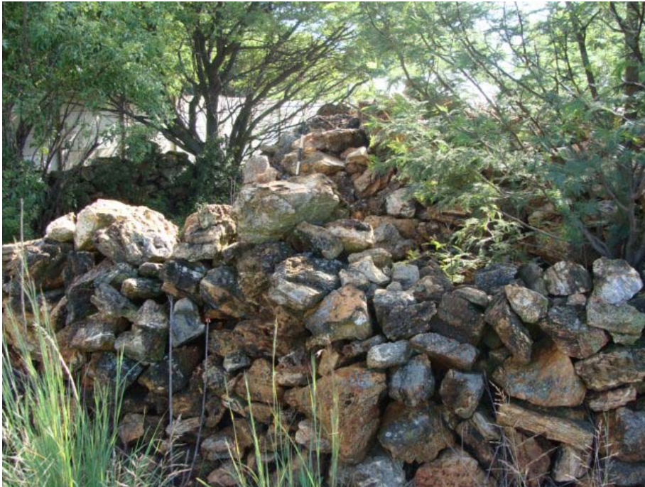
Figure 28 View of the platform on which the corrugated iron blockhouse stood and the stone wall surrounding it.
