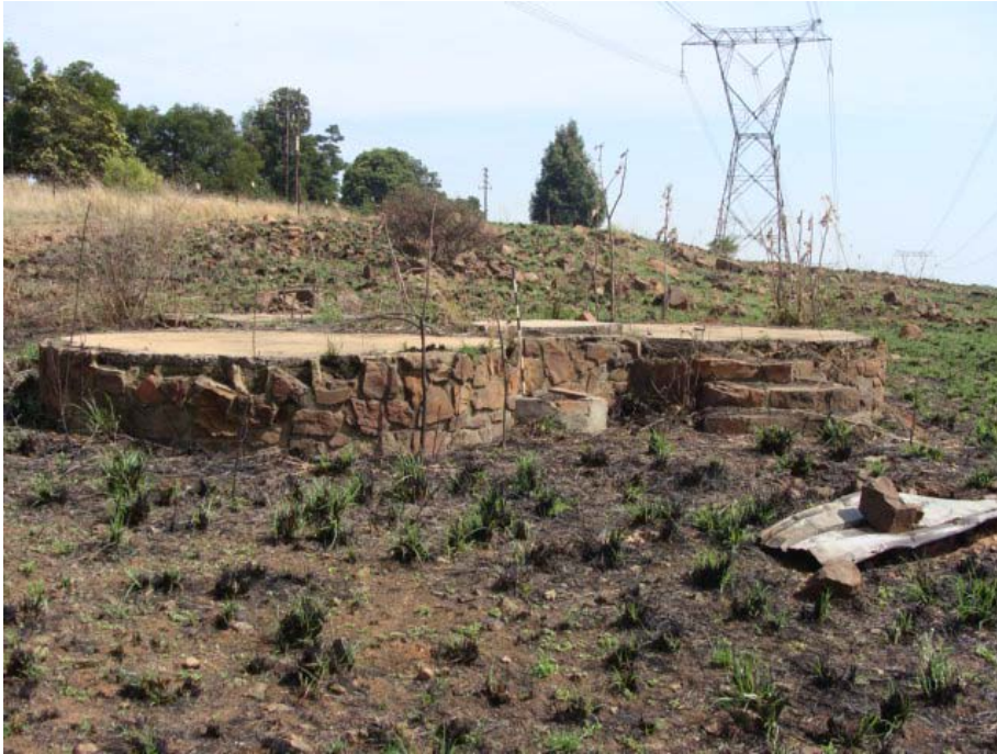
Figure 26 Foundations of the building numbered feature 9.
