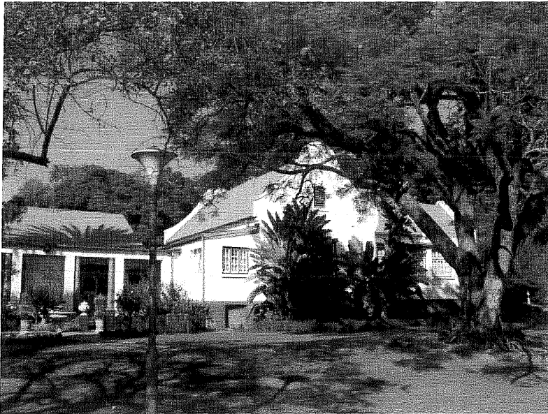
Figure 3 Northern façade of the Opstal
