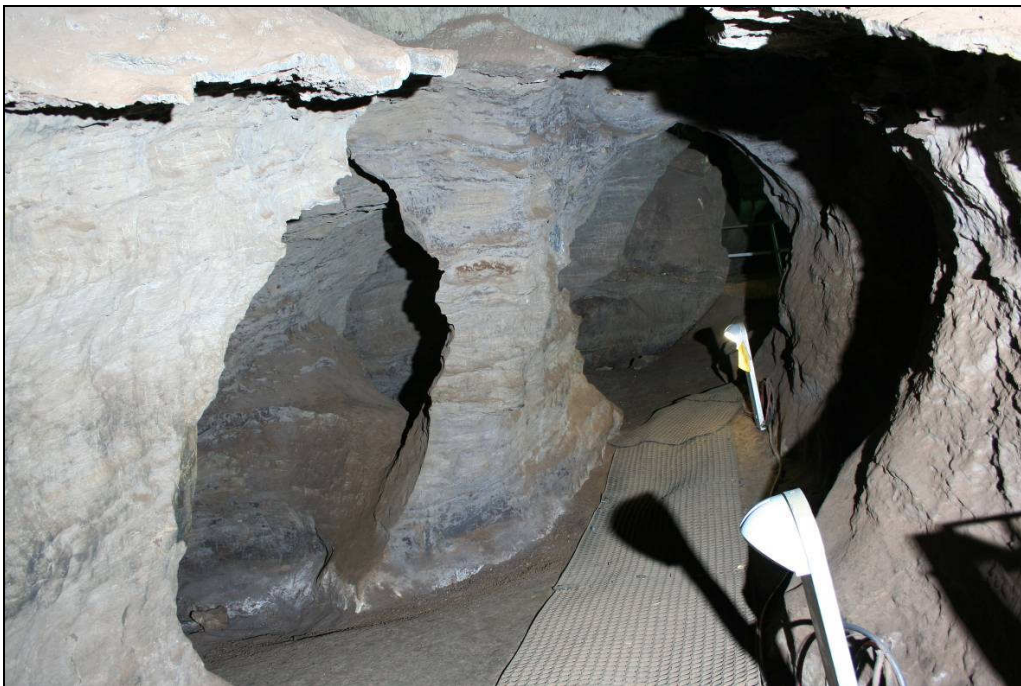
Figure 5 – Back of the rock wall on the Milner Hall side
