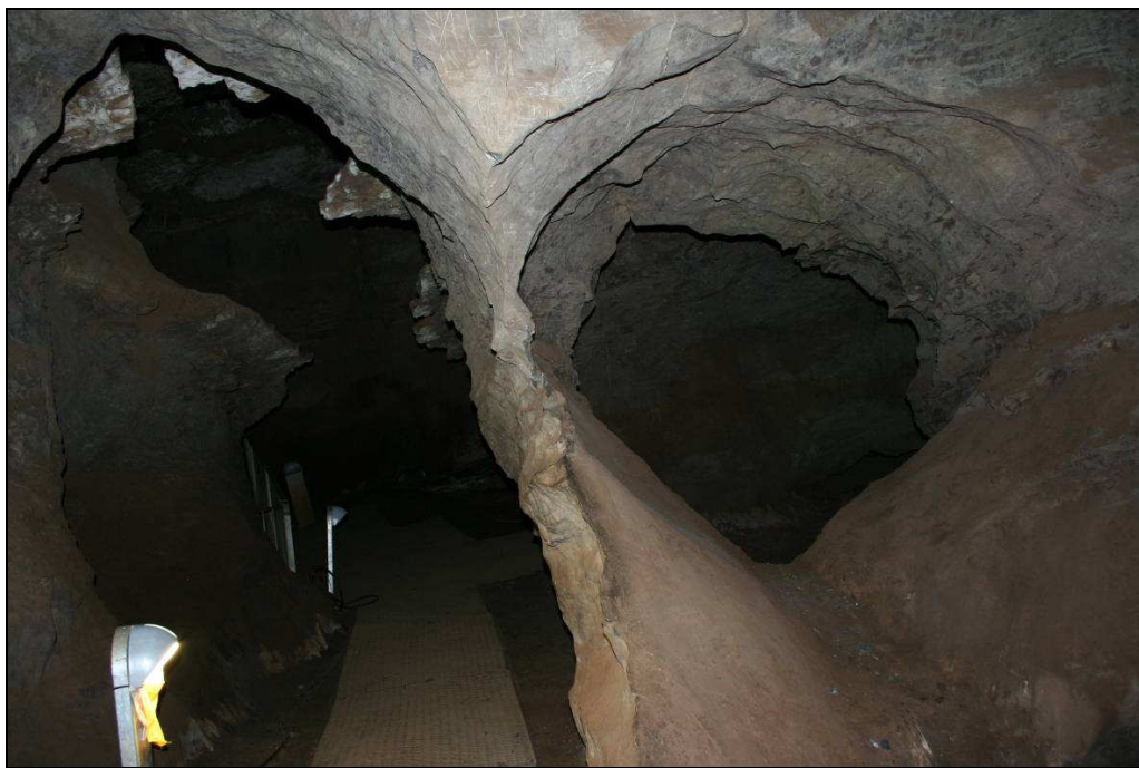
Figure 3 – Pillar of Rock indicating fracturing
