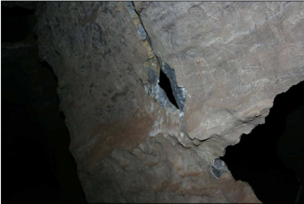
Figure 4 –Fracturing in rock wall
