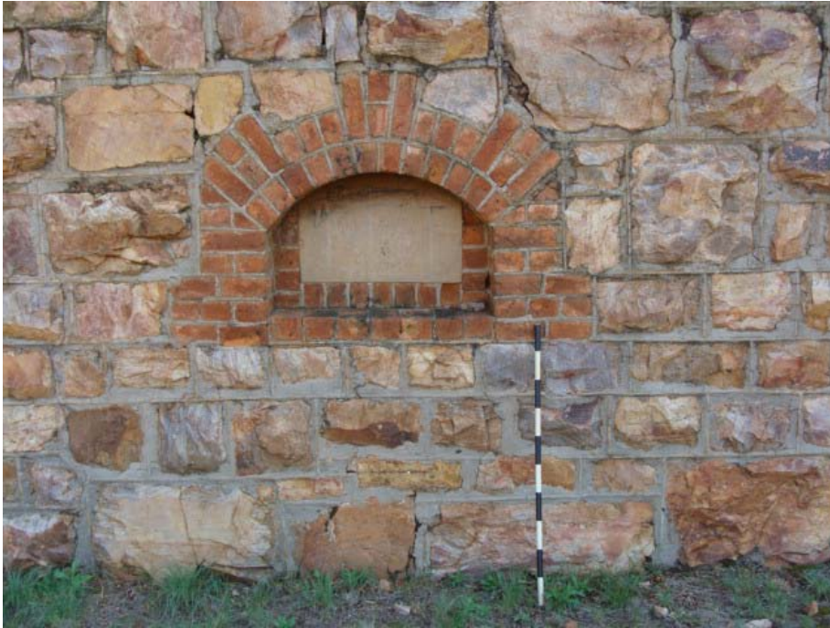
Figure 91 Loophole in the front wall of the fort. It was apparently closed by the former City Council of Pretoria.
