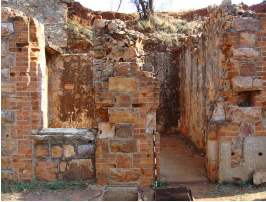
Figure 125 Front view of the hospital room at the fort.
