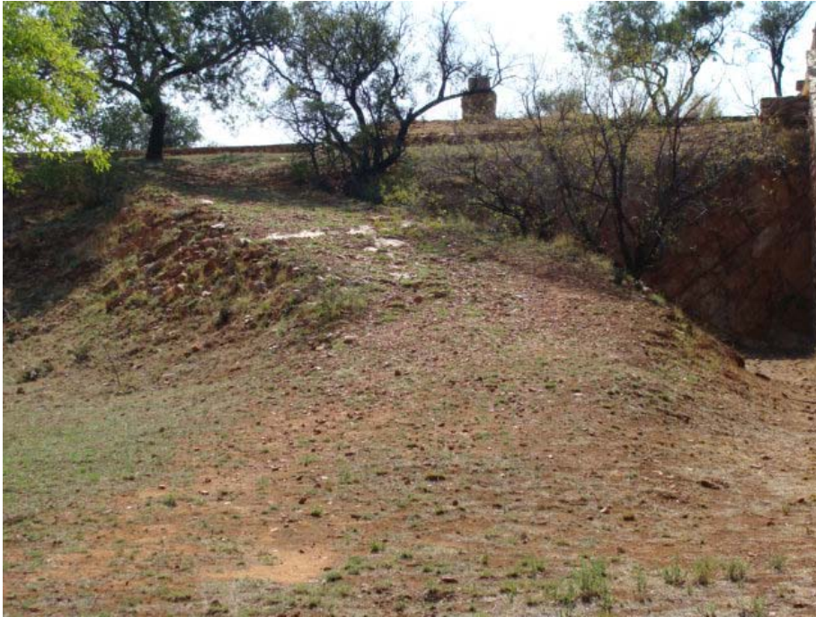
Figure 99 The ramp that gave access to the roof of the fort. It was used to move the canons to the roof. Also note the original rock face on the right hand side that was incorporated into the design of the fort.
