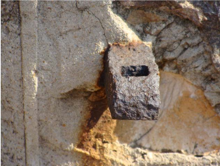
Figure 149 Window/ door latch at one of the rooms at the fort.
