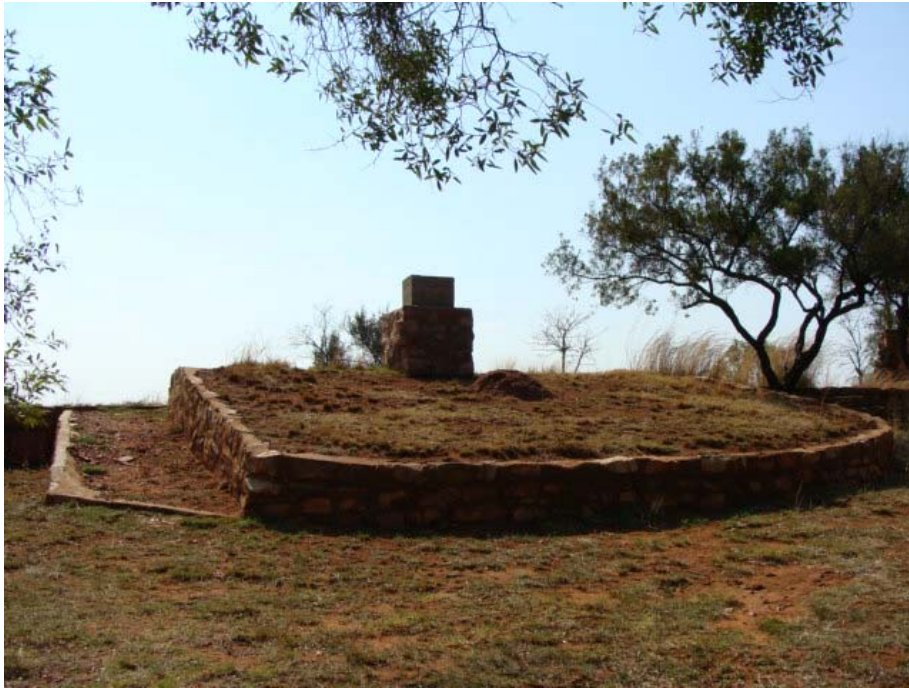
Figure 157 Stone walling on the roof of the fort which probably dates from a later period in time as the Anglo Boer War as the style differs from other stonework.
