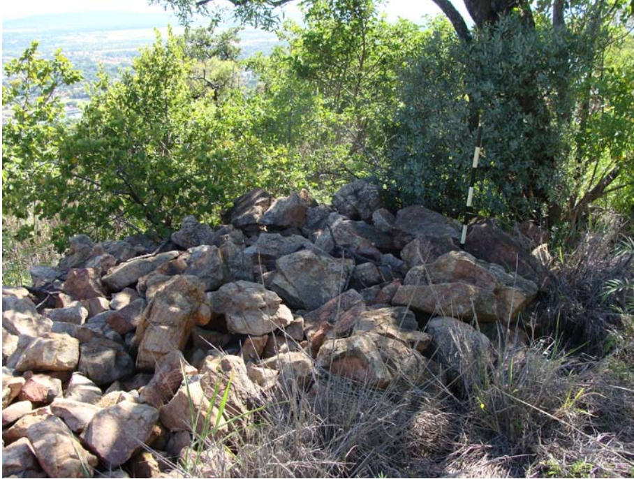
Figure 18 Stone wall at site no 3.
