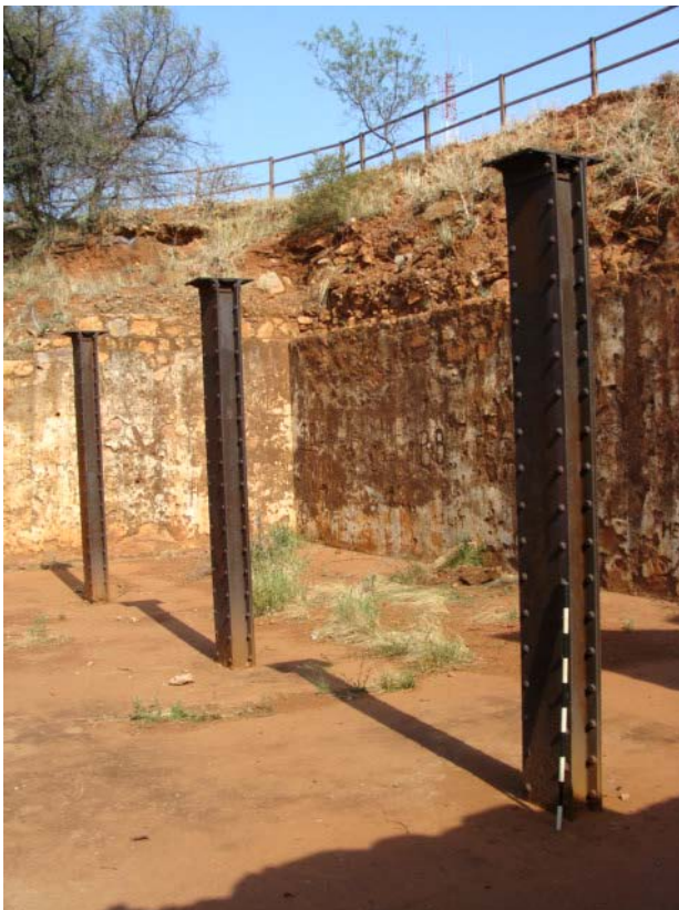
Figure 116 Steel pillars, like these ones in the sleeping quarters, were used to keep the concrete roof in position.
