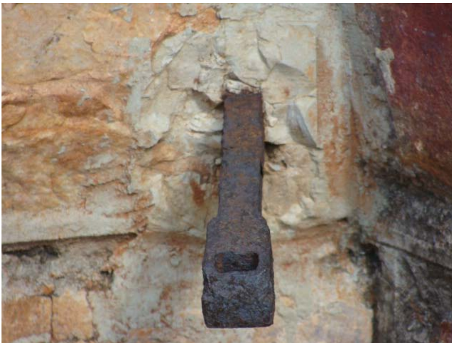
Figure 148 Window/ door latch at one of the rooms at the fort.
