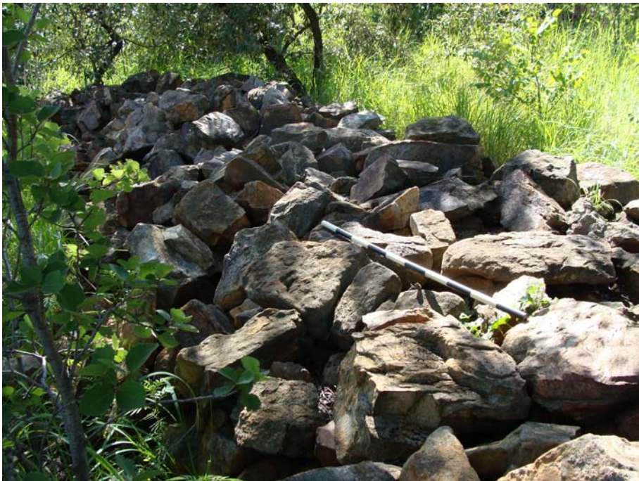
Figure 17 Another high stone wall at site no 3.
