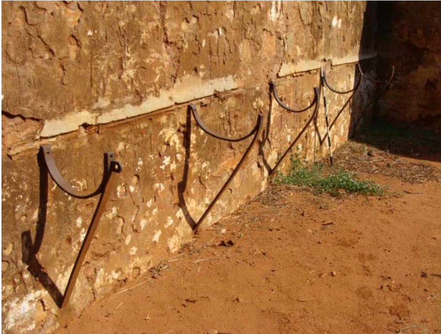
Figure 107 These metal arms are where the troughs were placed in the stable.
