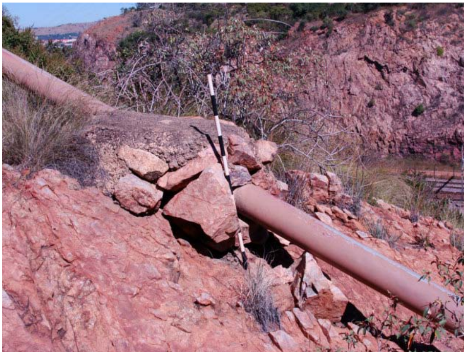
Figure 70 Pillar to keep water pipe serving the waterfall in position.
