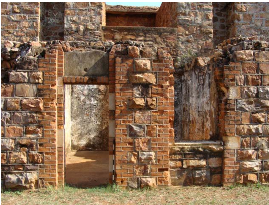
Figure 118 Front view of the machine room.
