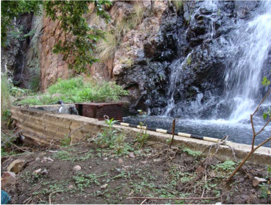
Figure 78 Catchment dam below the waterfall.
