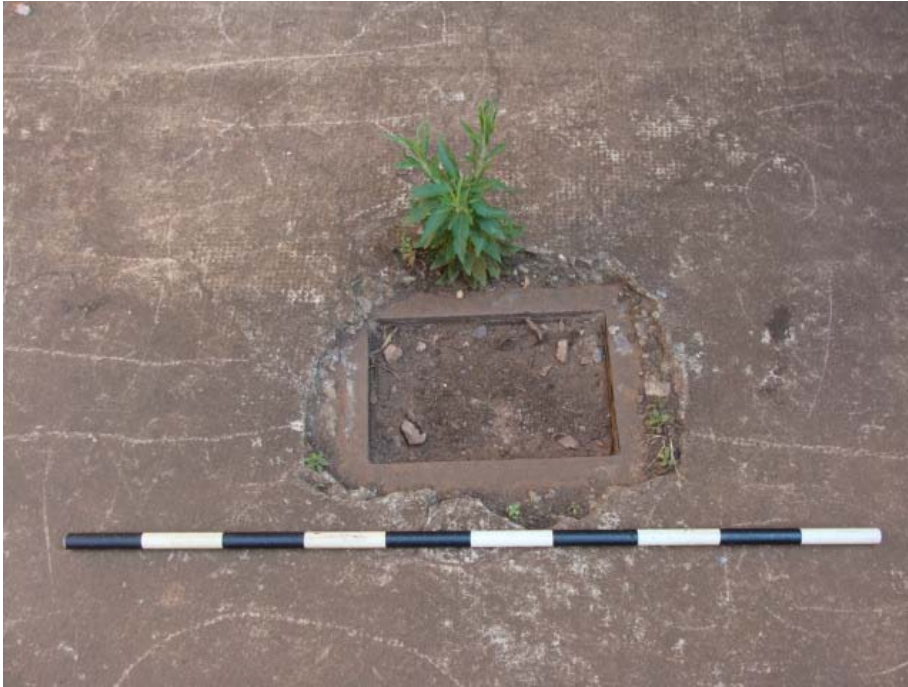
Figure 131 Place where the above steel pillar was removed from.
