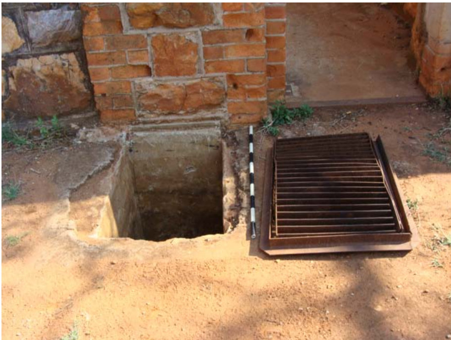
Figure 134 Original entrance to the water reservoir. The grid is a later addition, but even this was vandalized.
