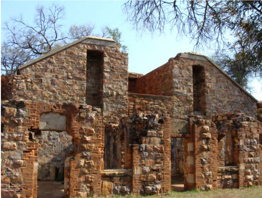
Figure 153 Close up view of the storage area for canons.
