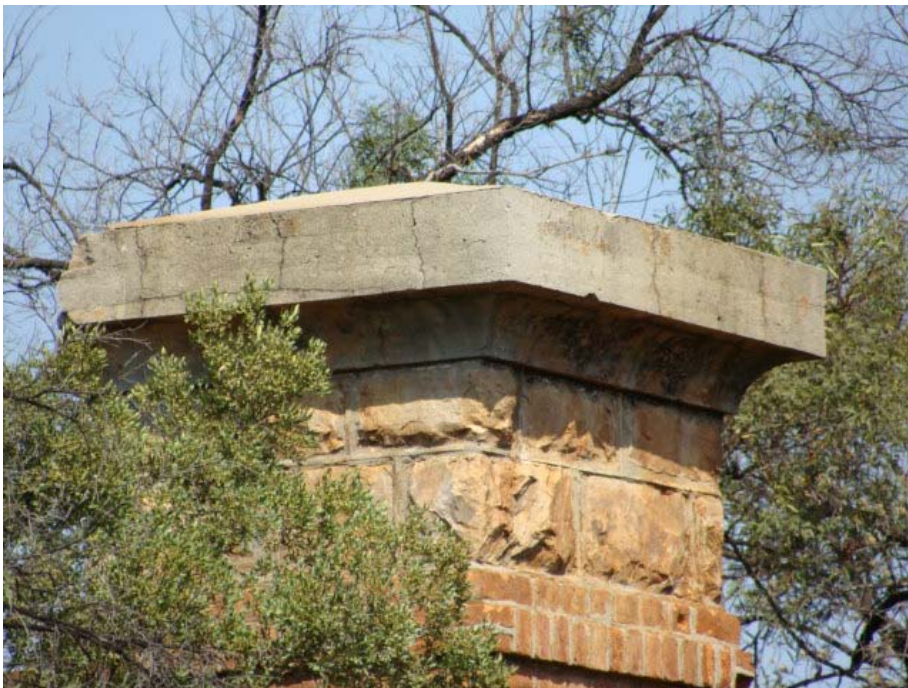
Figure 88 Pillar at the entrance to the fort.
