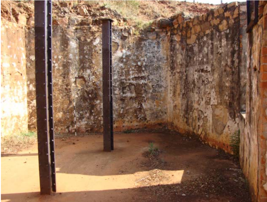
Figure 113 Inside of the provisions store room at the fort.
