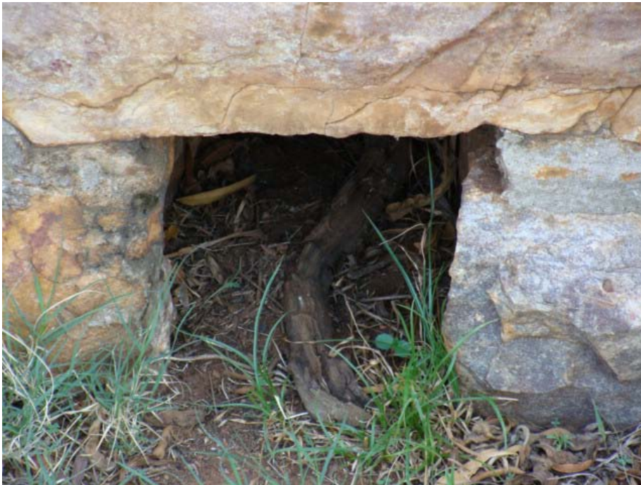
Figure 138 Water outlet in the outside wall of the fort.
