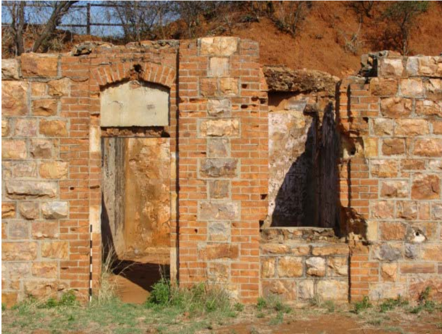
Figure 109 Front view of the officers' room.
