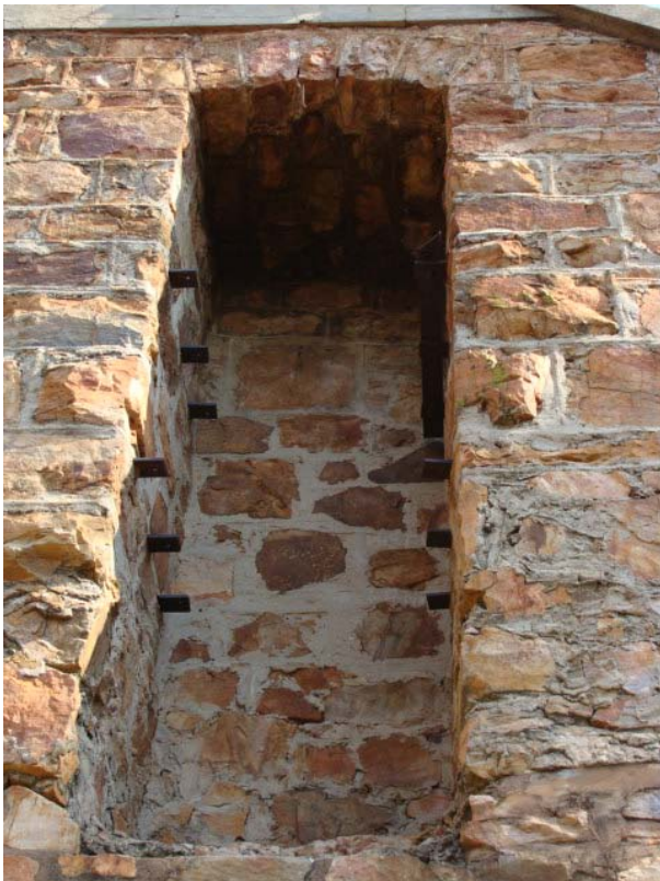
Figure 156 Another view of the storage niche for first line ammunition. Note one of the metal bars of the shelves are still in position.
