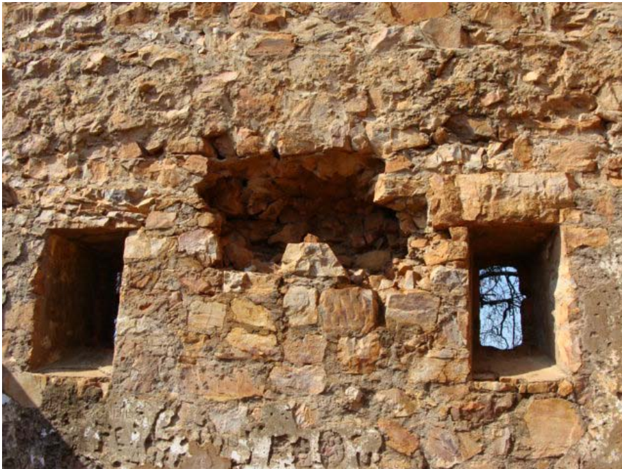
Figure 108 Windows at the stable.
