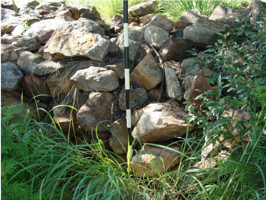
Figure 16 High stone wall at site no 3.
