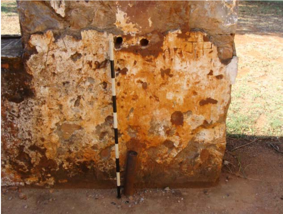
Figure 123 Inside of the telegraph room. The steel pipe was used to protect the electric wiring.
