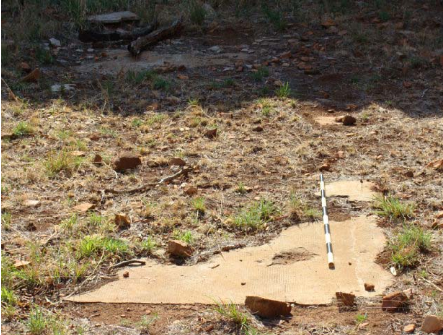
Figure 151 Another view of the floor indicated. Note the damage on its furthest side.
