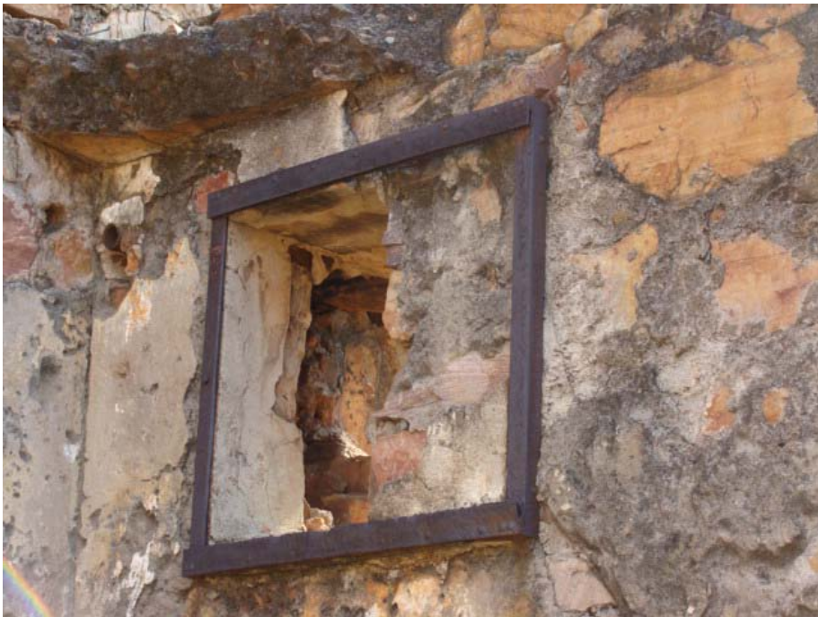
Figure 144 Ventilation shaft with frame for sliding blind still attached to it.
