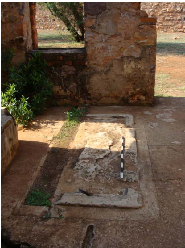
Figure 120 Another view inside of the machine room in the fort. Note the area where the generator possibly was attached.
