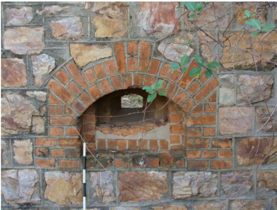
Figure 92 Open loophole in the front wall of the fort.
