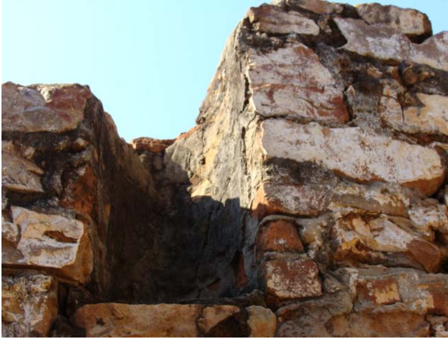
Figure 143 Ventilation shaft in one of the rooms at the fort.
