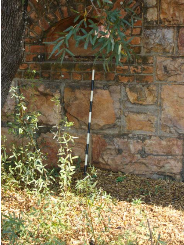
Figure 139 Small furrow running from a water outlet away from the fort.
