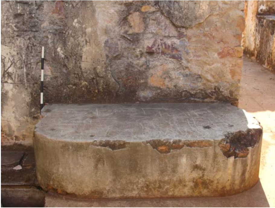
Figure 121 Another view inside the machine room.
