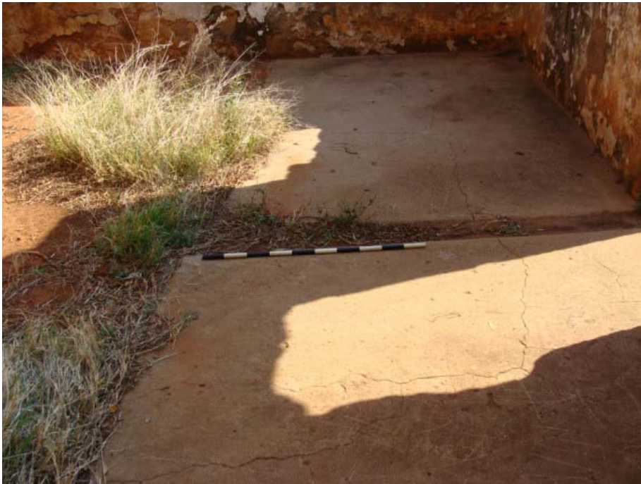
Figure 106 Water furrow inside of the stable at the fort.
