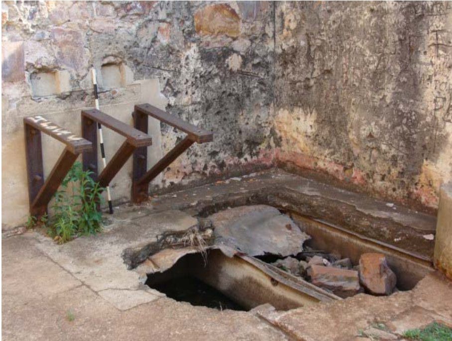
Figure 119 Inside of the machine room at the fort. The steel arms were used to place heavy machinery on and the reservoir beneath the floor was probably used for paraffin.
