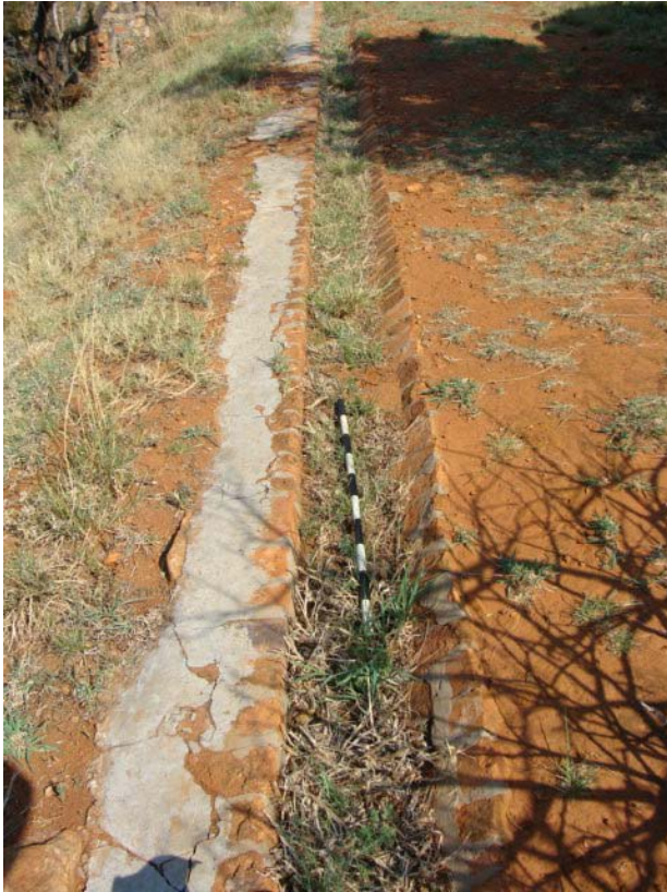
Figure 141 Water furrow on the roof of the fort.
