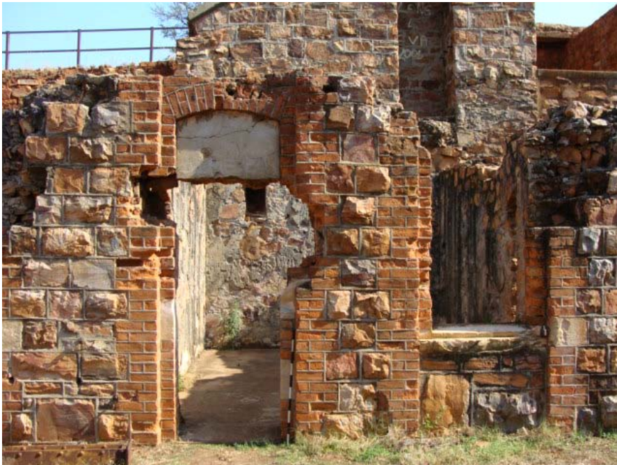
Figure 124 Front view of the kitchen room at the fort.
