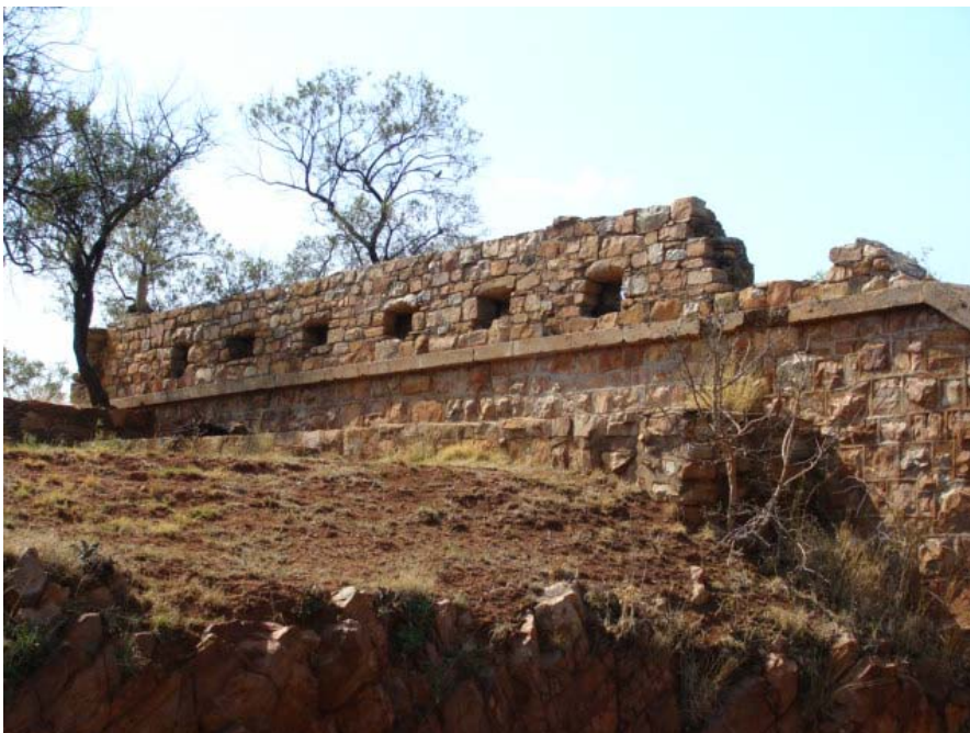
Figure 96 This wall on top of the fort wall was probably built by the British after they took over the fort as the style clearly differs from the rest of the building.
