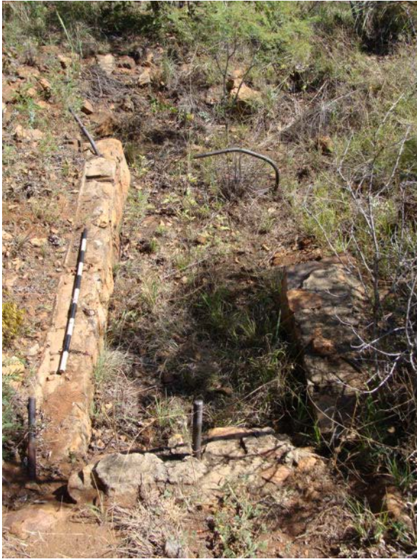
Figure 74 Concrete construction behind the fort which was probably used to fix large machinery on.
