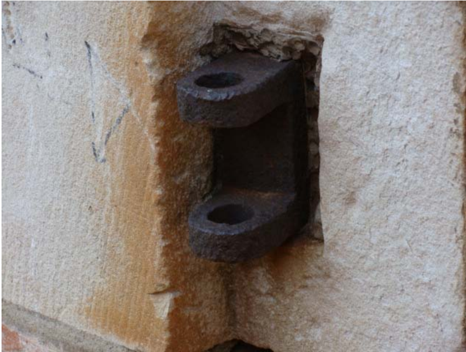
Figure 147 Window/ door hinge at one of the rooms at the fort.
