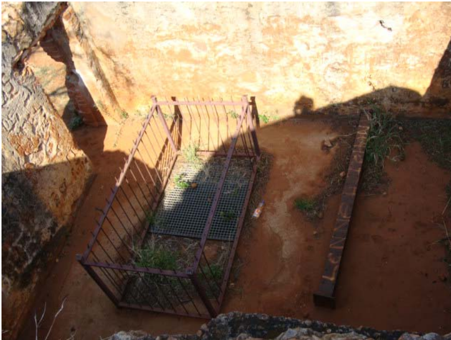
Figure 132 The water reservoir is beneath the ammunition store room. The floor of the ammunition room was damaged by someone trying to gain access to the reservoir. A barrier was erected to make the area safe, but even this was vandalized.
