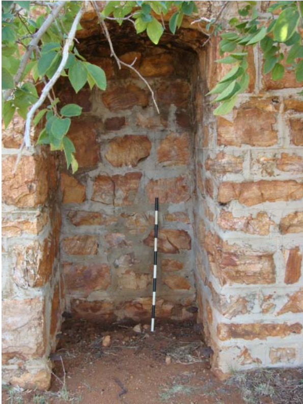
Figure 155 Storage niche for first line ammunition.
