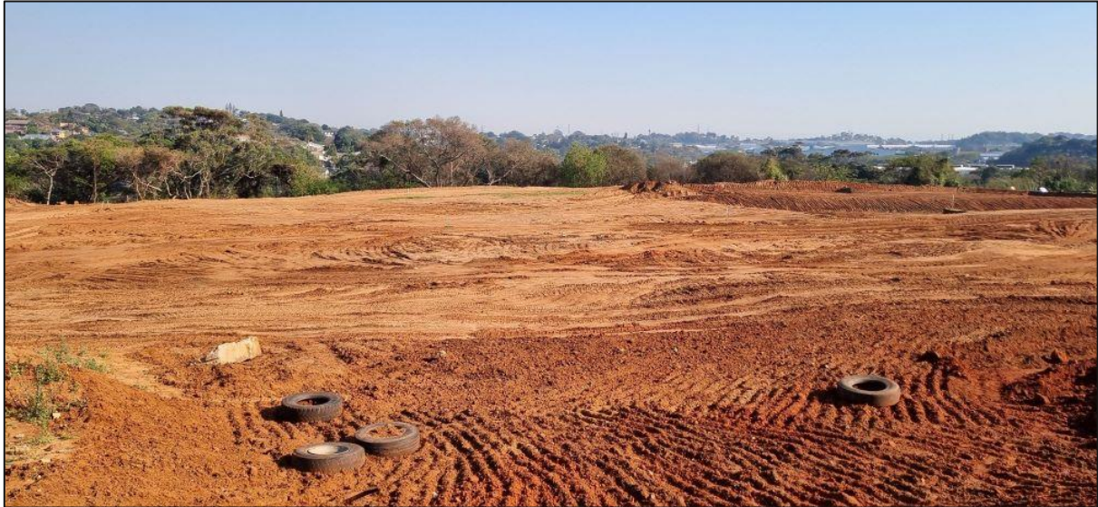
Plate 1: Photograph showing an overview of the project site where vegetation clearing and stripping of topsoil and subsoil has occurred.
