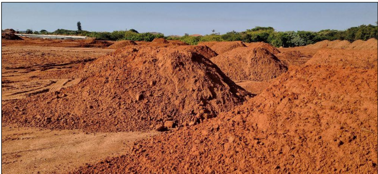
Plate 3: Photograph showing topsoil and subsoil stockpiles on the project site.
