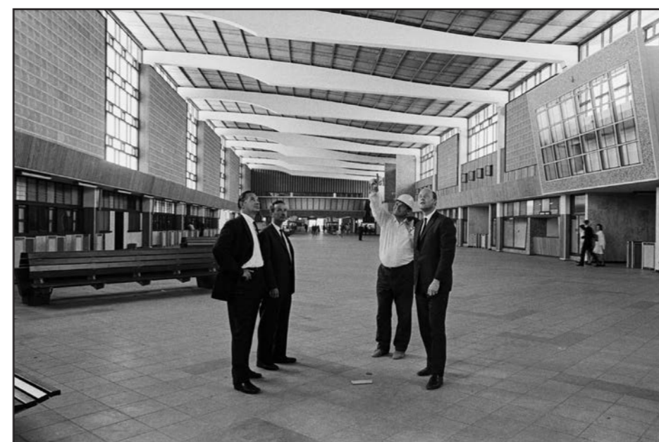
Figure 10: Inspection of the station concourse, showing the reinforced concrete sweeping “s” beams along the roof (source: SANL, Cape Times Collection)
