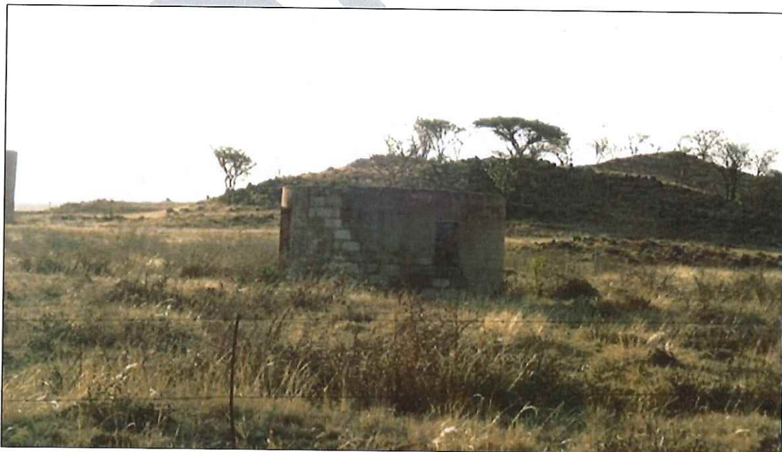
Figure 35: Site 009 Concrete bungalow
