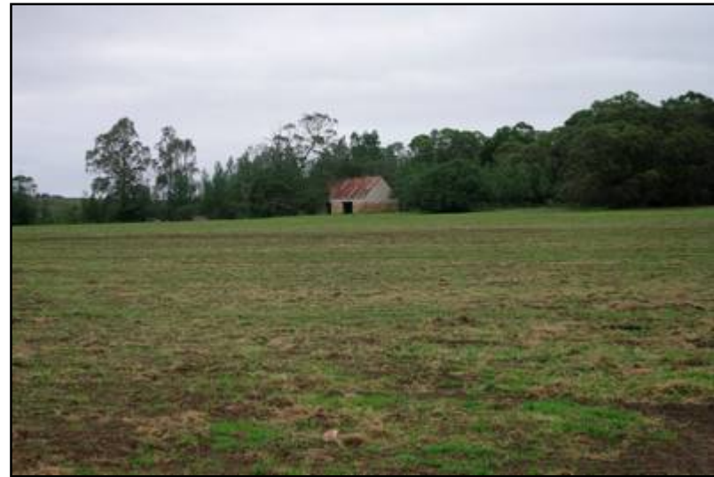
Plate 20: General view of the TBP-5.S1 Colonial Period infrastructure
