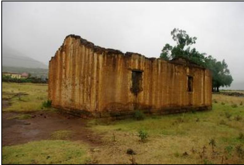
Plate 9: View of Site SSD-S2 with a livestock enclosure in the background [1]
