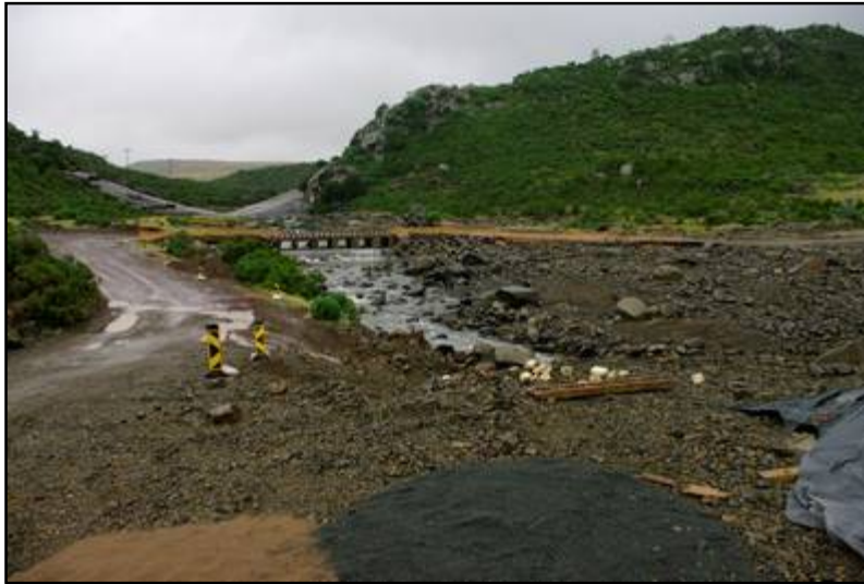
Plate 1: View of the temporary crossing structure across the Silver Stream
