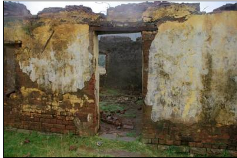
Plate 11: Close-up of the Site SSD-S2 entrance
