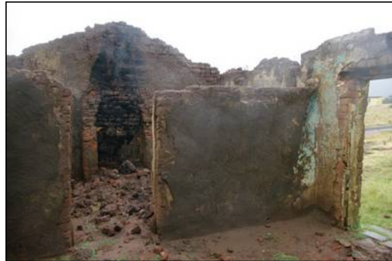
Plate 12: Interior view of Site SSD-S2
