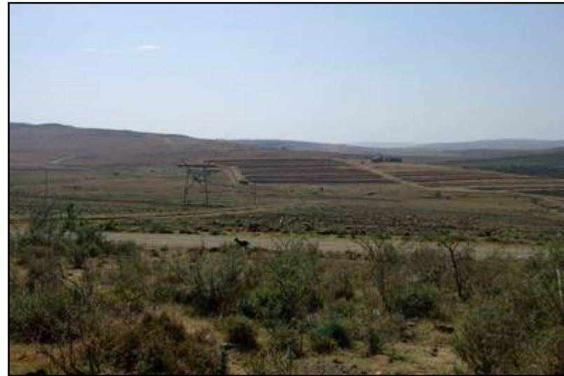
Plate 12: General view of the Tyalara to Qunu line route [3]
