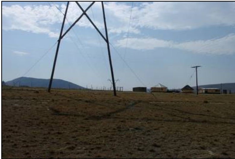
Plate 10: General view of the Tyalara to Qunu line route [1]
