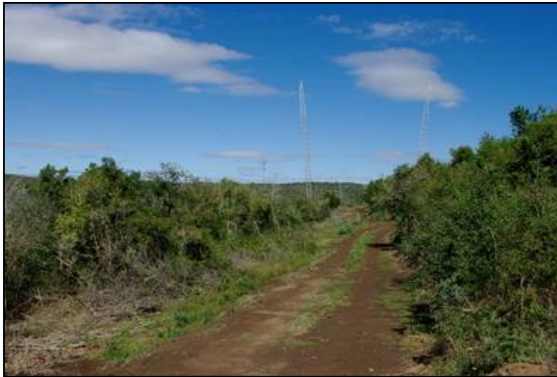
Plate 6: General view of the Neptune to Chaba line route [5]
