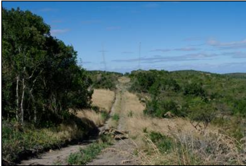
Plate 5: General view of the Neptune to Chaba line route [4]
