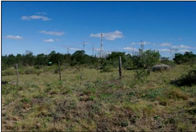
Plate 1: View of the Neptune substation
