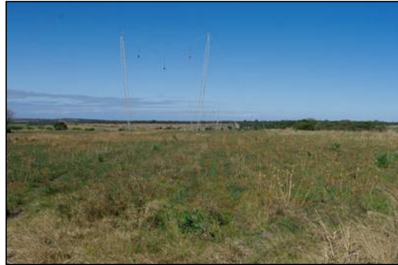
Plate 7: General view of the Neptune to Chaba line route [6]
