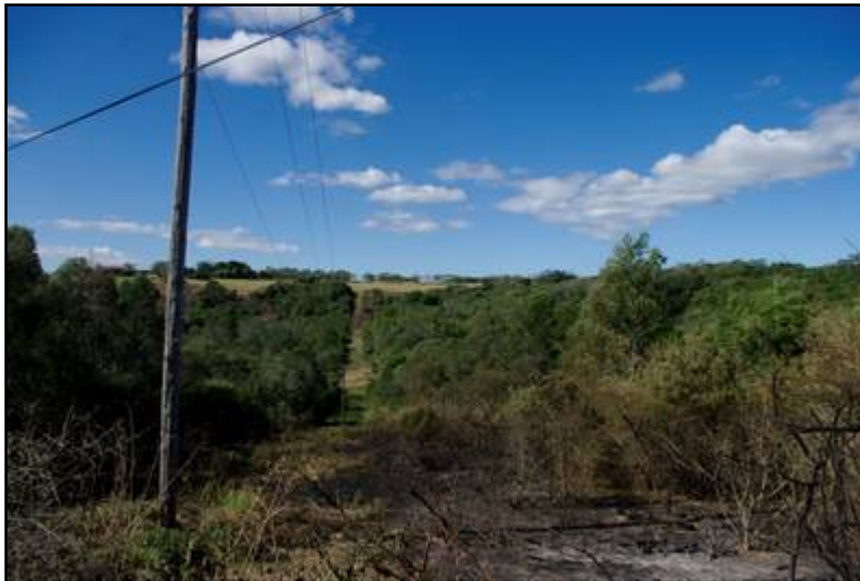
Plate 2: General view of the Neptune to Chaba line route [1]
