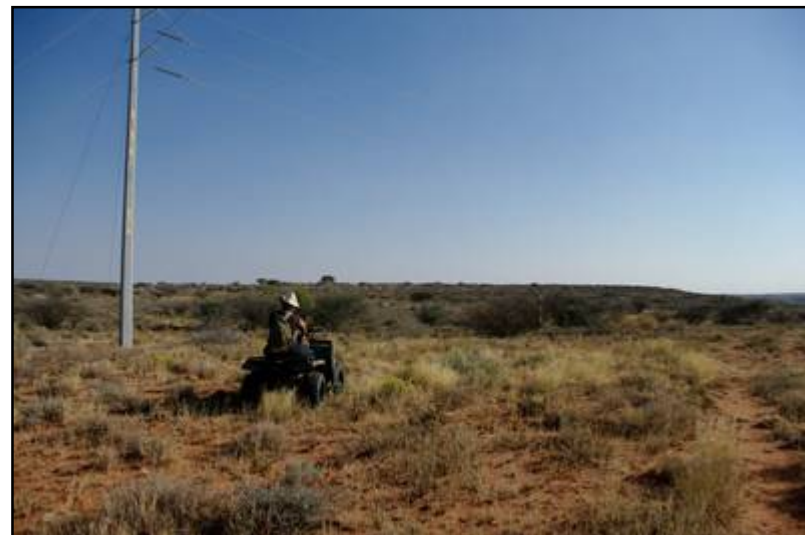
Plate 12: View of the Option A power line from the existing substation
