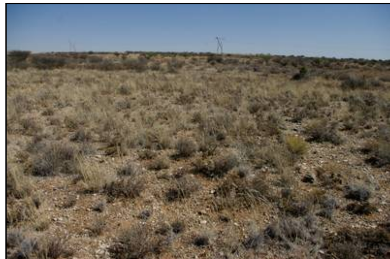
Plate 16: The Option B power line in the vicinity of the new substation
