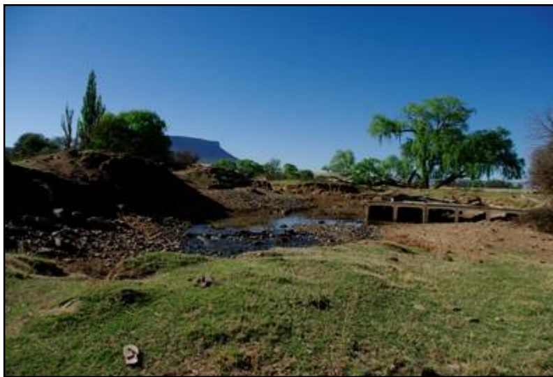
Plate 1: General view of the Becclesfarm Bridge – Site 1 study site [1]
