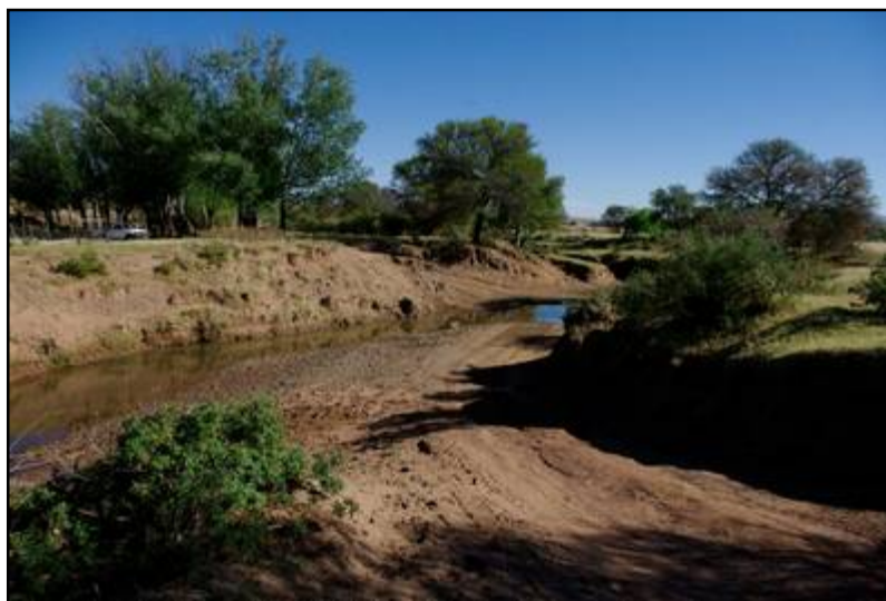
Plate 4: General view of the Becclesfarm Bridge – Site 2 study site [2]
