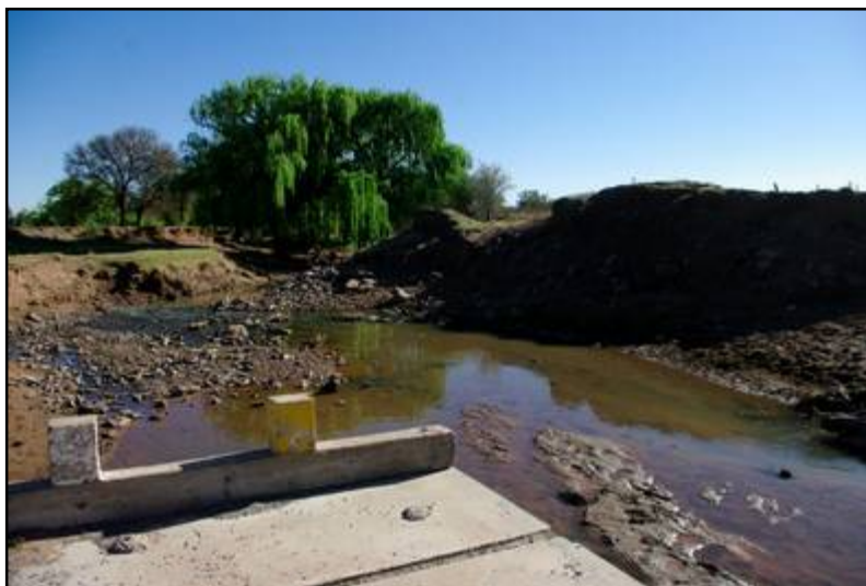
Plate 2: General view of the Becclesfarm Bridge – Site 1 study site [2]
