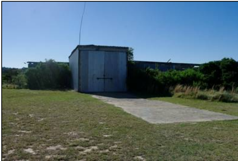
Plate 2: Close-up of structure KG-C1
