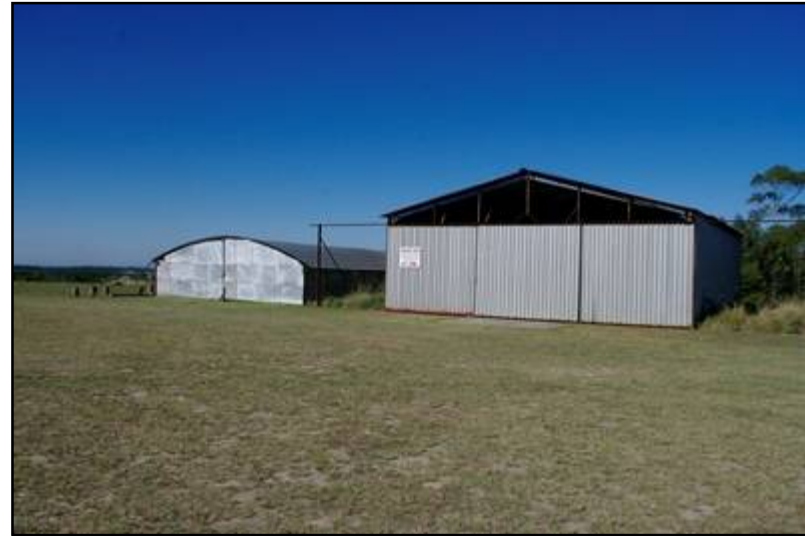
Plate 3: Close-up of structure KG-C2
