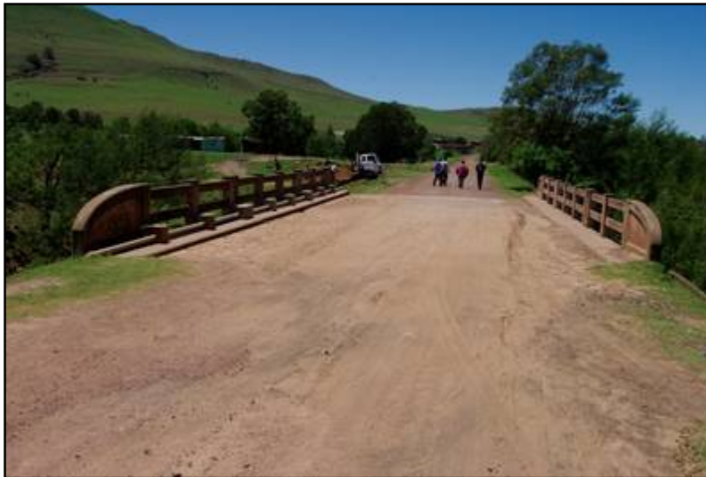
Plate 6: View of the contemporary MRD-1 bridge [1]
