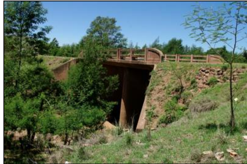
Plate 7: View of the contemporary MRD-1 bridge [2]
