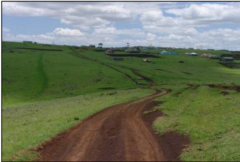
Plate 2: General view of the pipeline, running adjacent to the access road
