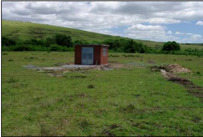
Plate 1: View of the pipeline at the Ngcizele borehole
