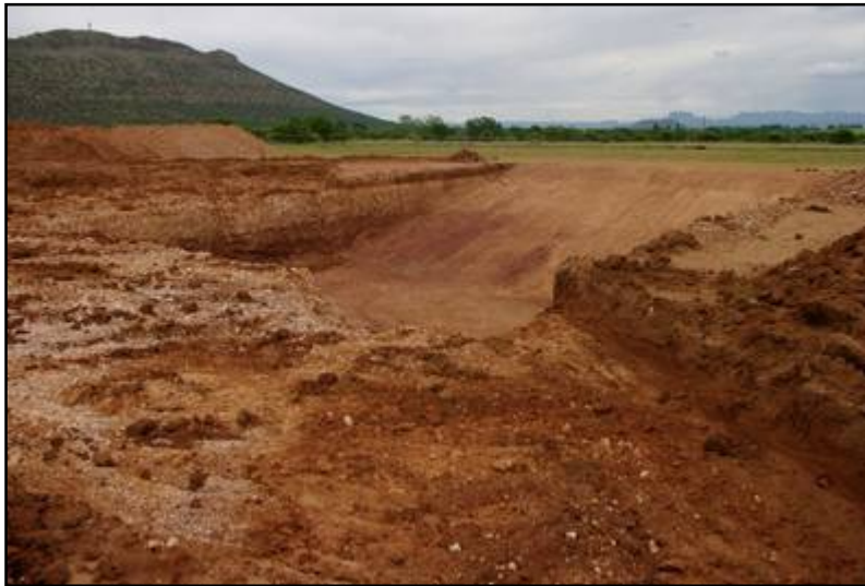
Plate 6: General view of the 2 nd foundation excavation
