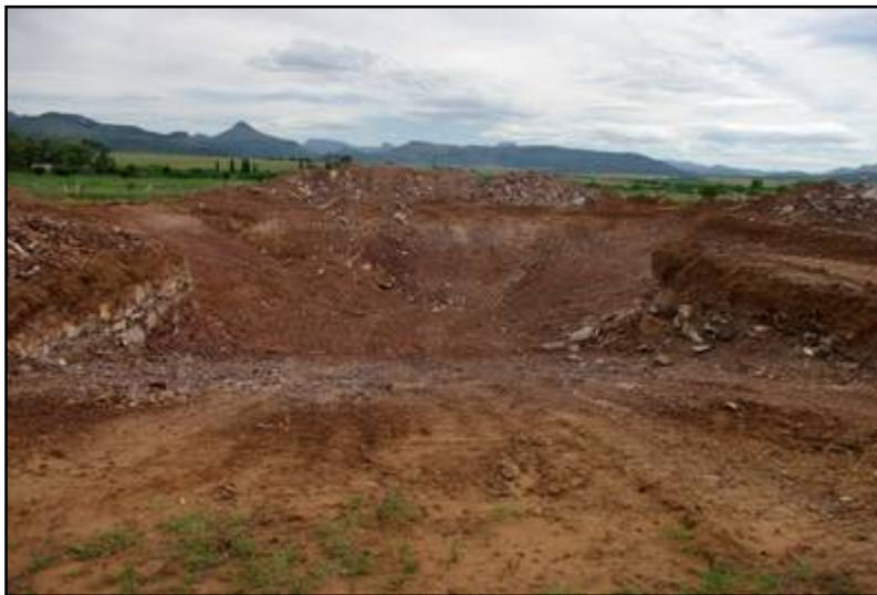
Plate 2: General view of the 1 st foundation excavation
