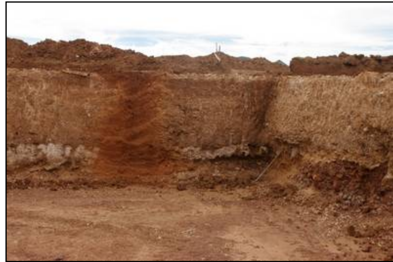
Plate 7: General view of the 3 rd foundation excavation
