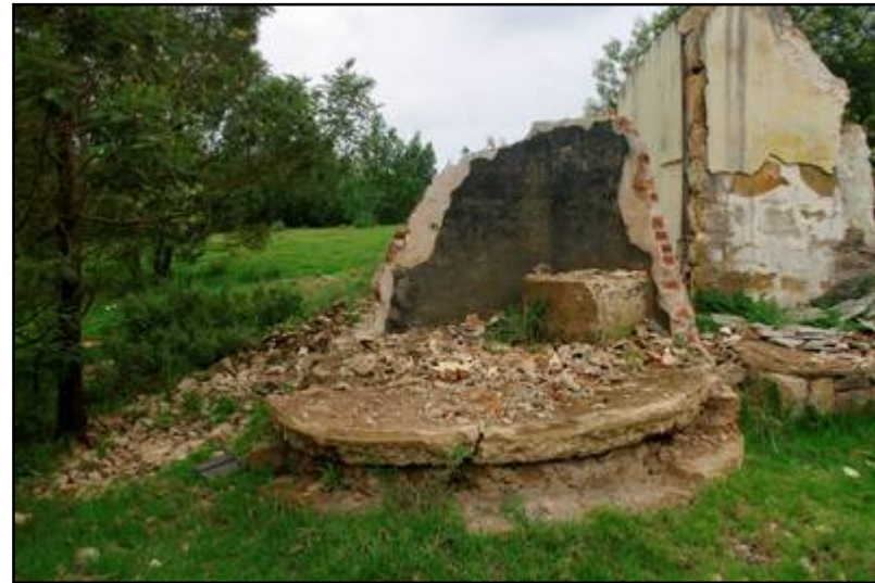
Plate 8: The later addition brick and cement water tank at Site MEL08
