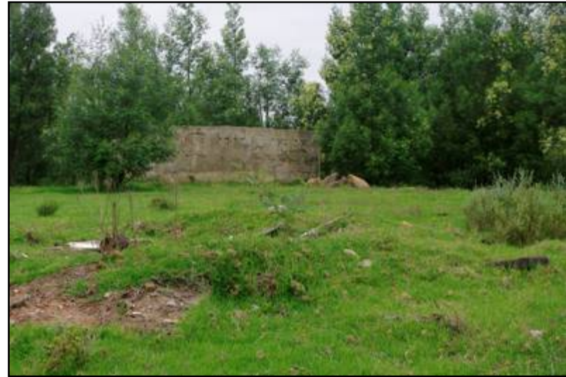
Plate 7: An old cement dam in close proximity to the structure ruins
