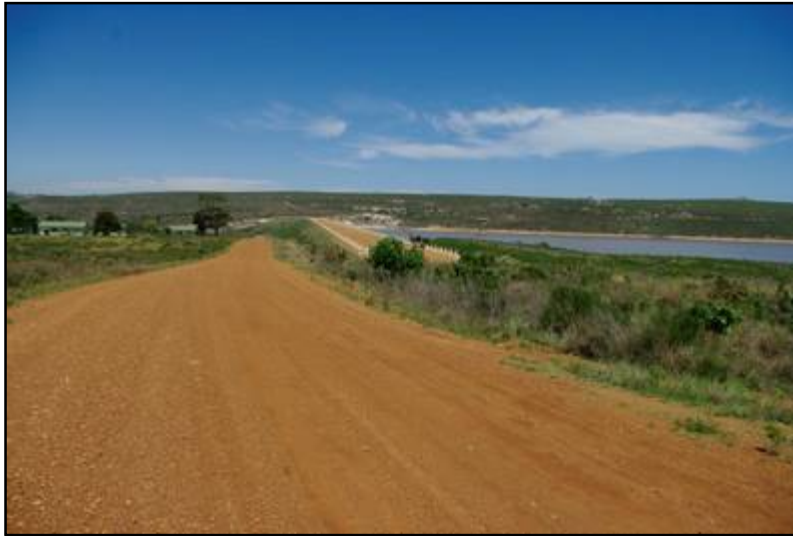
Plate 17: General view of the Impofu dam wall area
