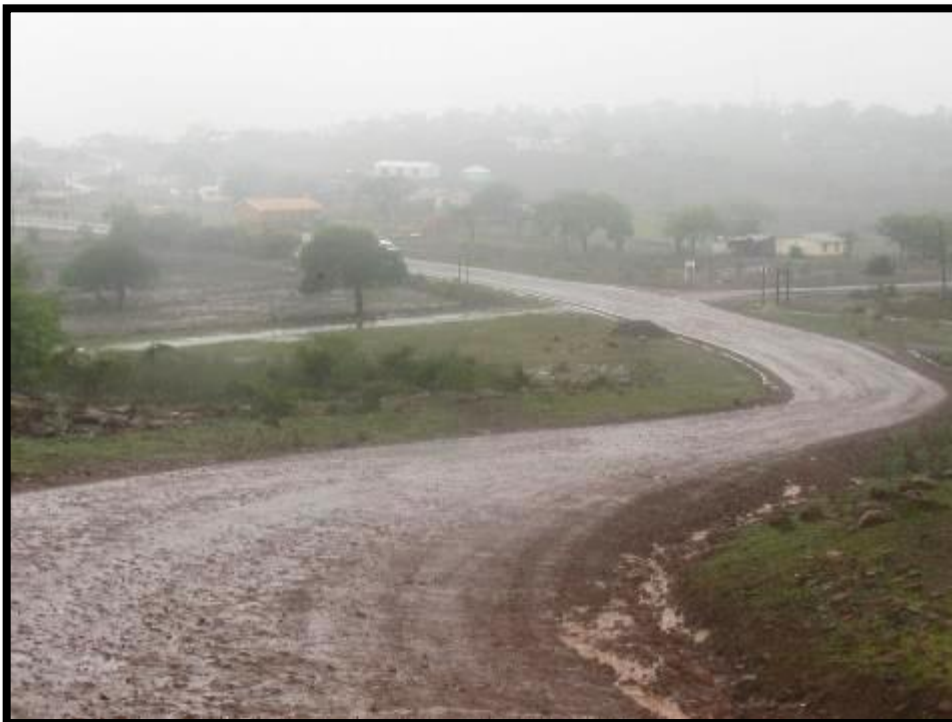
Figure 6. Southern section of the P236 near Ubombo.
