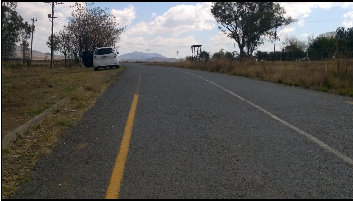
Plate 1: Road currently being used
